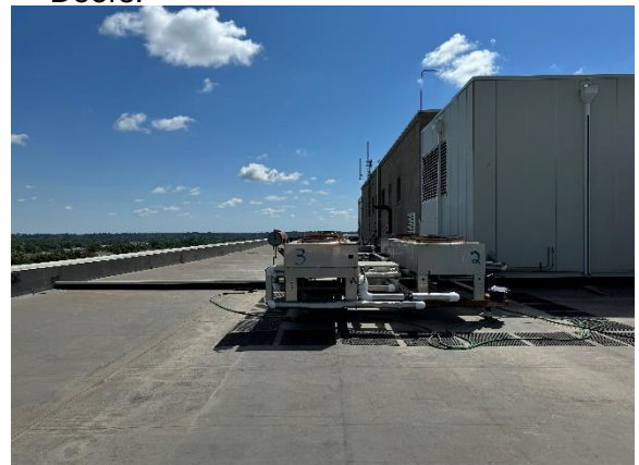
Photo #6 View of HVAC units to be removed.
