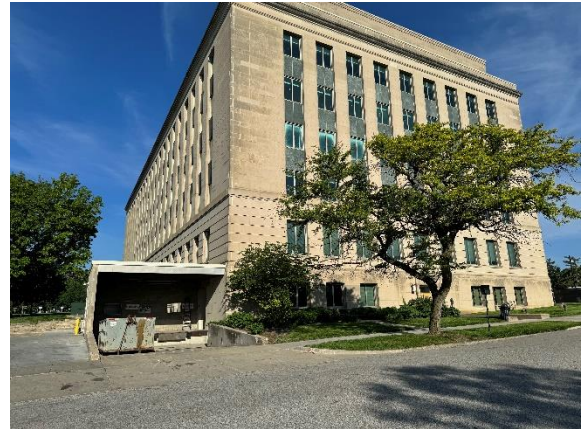
Photo #2 View of the loading dock on Lucas Building
