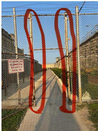
Gate section to be removed by ASP
