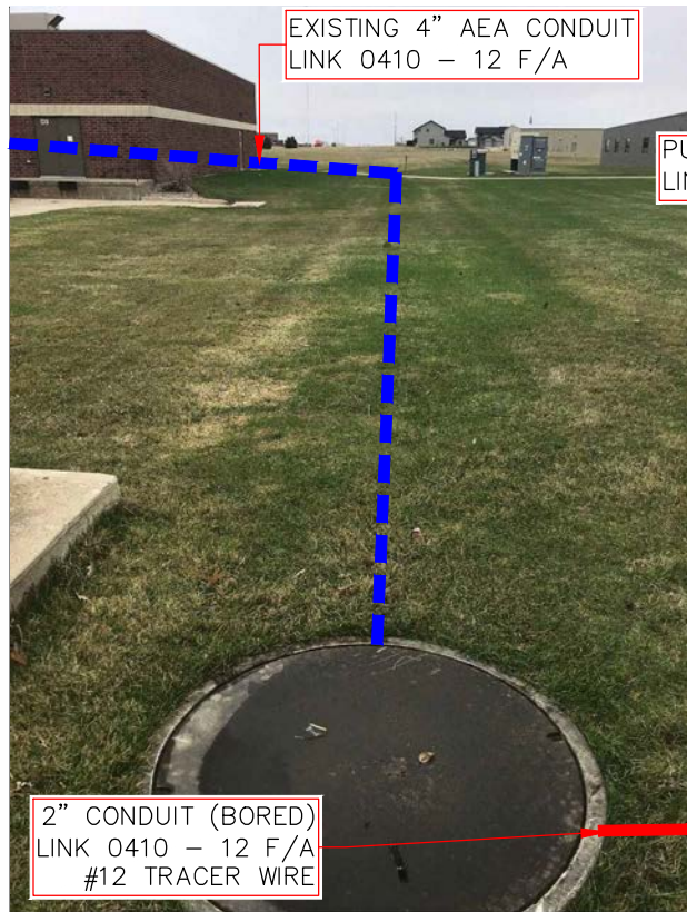
11.1 EXISTING HANDHOLE 48" ROUND LOOKING EAST STA. 42+35
