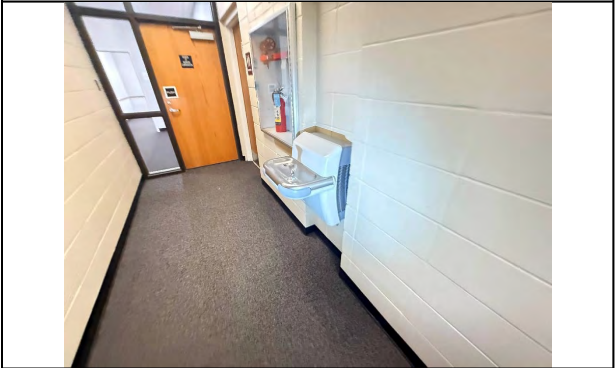
Photo 13: View of a fire extinguisher, a water fountain, and an automatic door closer present on site.
