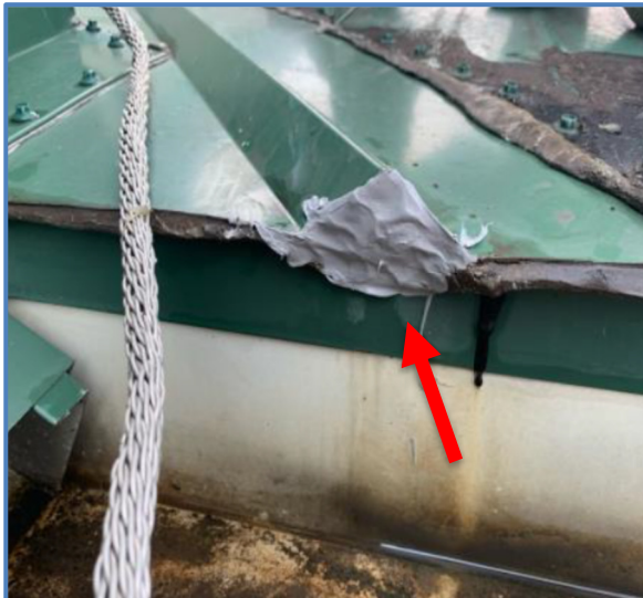
Photo 58: Temporary repair was completed by Tremco while onsite to prevent further bulk water intrusion at this location.
