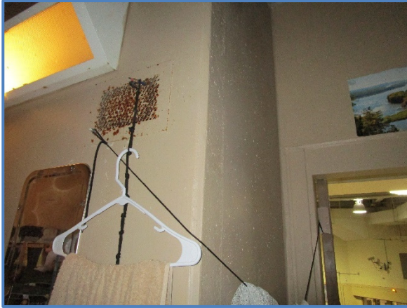
Photo 1: Ducted supply grilles in the cells have rusted, likely the result of condensation occurring on the cold surface.
