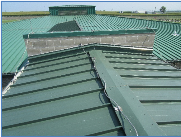
Photo 32: The CMU block wall located at the fire wall separating the Pod from the main building where 1 of 3 RILEM Tube tests were conducted. RILEM tubes are filled with water and situated to drain through the masonry; water levels in the tubes are checked every 5 minutes over a 20-minute period. An acceptable performance is achieved if the level of water drops no more than 20% of the original height during the 20-minute test period.
