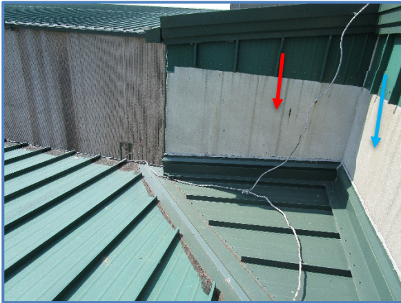
Photo 34: RILEM tube test location #2 (Red Arrow) was located on the smooth precast wall panel. RILEM tube test location #3 (Blue Arrow) was located on the rougher precast wall panel.
