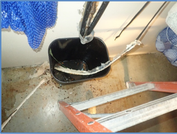
Photo 61: The trashcan filled quickly from the nozzle test around the valley pan.
