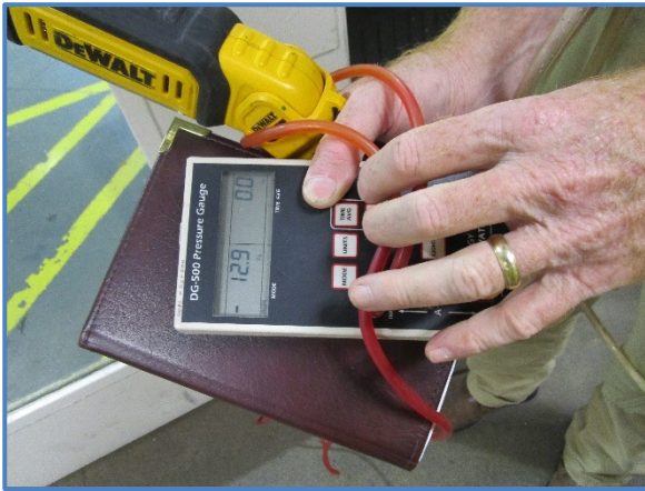
Photo 20: A digital manometer measured the negative pressure between Unit 1 of Pod-C and the common hall area to be -12.9 Pascals. This is a significant negative pressure resulting from an unbalanced HVAC system. This will cause outside air and moisture to be sucked into the occupied conditioned space.
