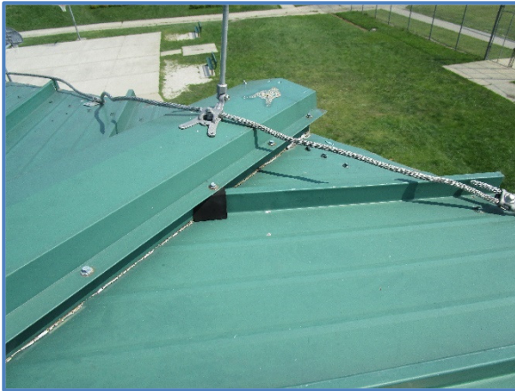
Photo 36: North corner of Pod-C, Unit 2, where the invasive inspection of the roof assembly was conducted to determine the actual construction of the roof assembly.
