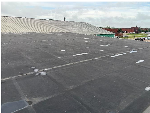
Photo #5 Roof of North Freezer (No Asbestos Containing Materials Found)
