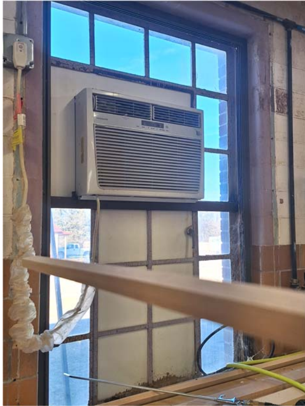
INTERIOR STEEL WINDOW WITH AC
