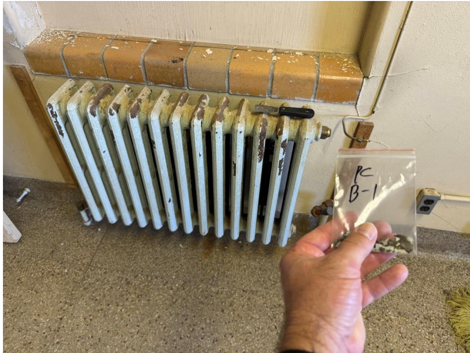
View of the Teal Lead Containing Paint. (PCB-1, 0.42% Pb)
