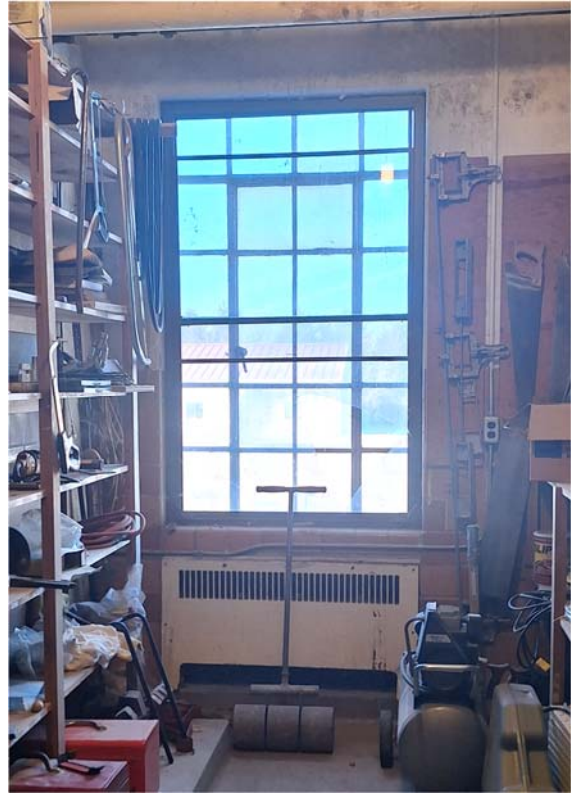
INTERIOR STEEL WINDOW WITH RADIATOR
