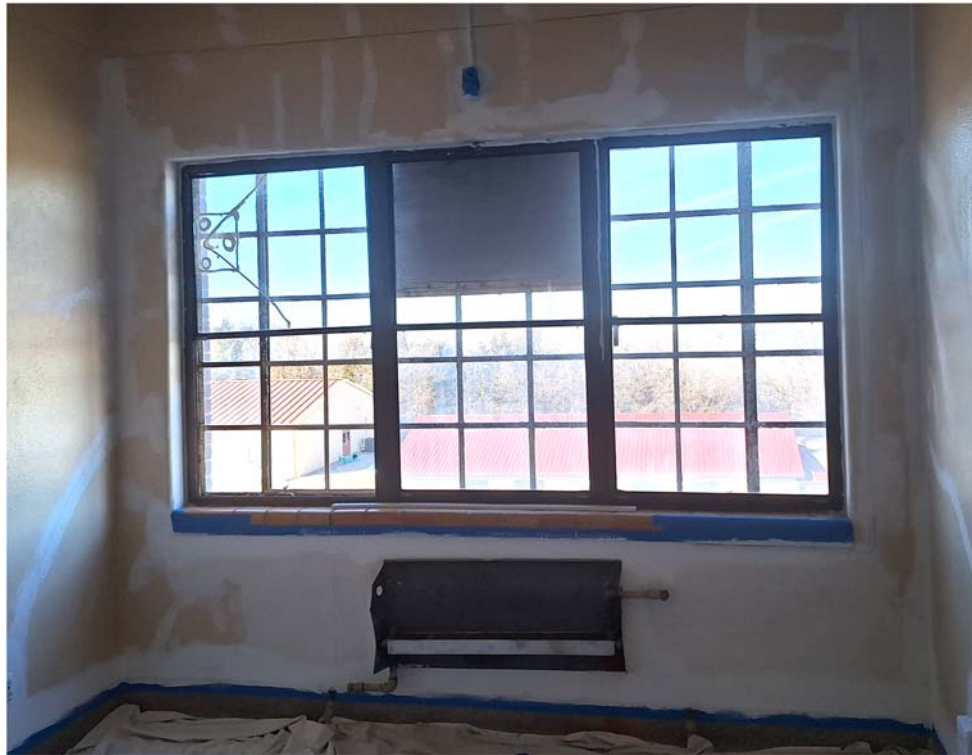
INTERIOR 3RD FLOOR - EXISTING TRIPLE STEEL WINDOW
