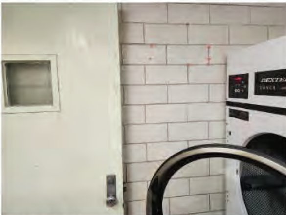
Photo #17 View of lead containing white and beige 6-inch by 4-inch glazed ceramic block.
