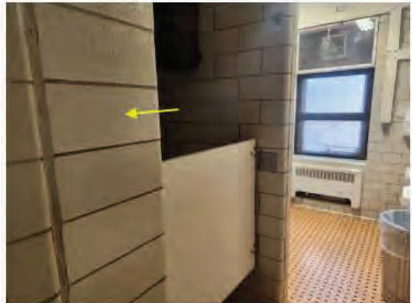
Photo #16 View of lead containing white and beige 6-inch by 4-inch glazed ceramic block.
