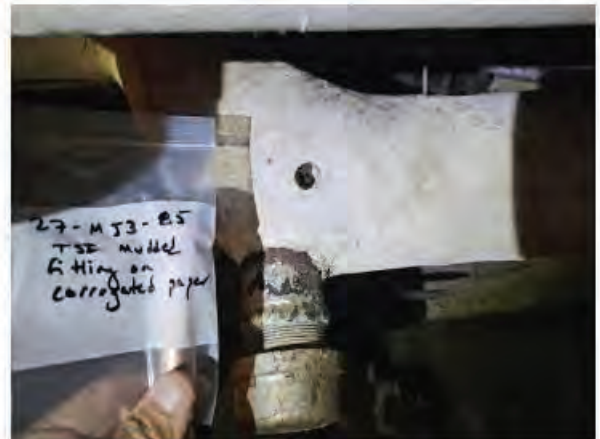
Photo #10 Photo of asbestos containing TSI mudded fitting on corrugated paper pipe insulation, HA 27.
