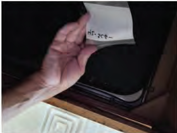
Photo #13 Photo of asbestos containing white and black sink undercoat, HA 42.
