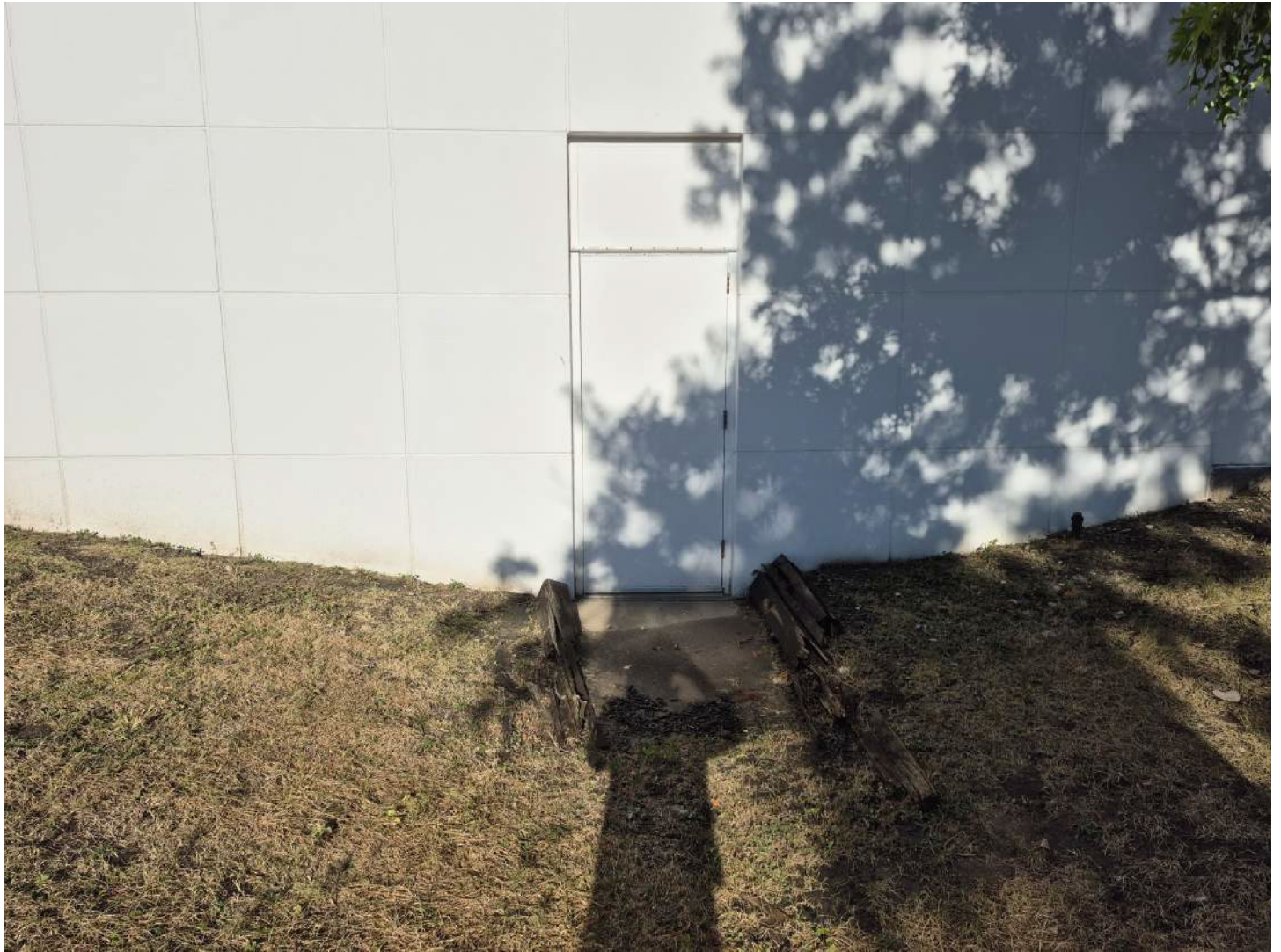
Existing Auditorium exit door, retaining walls and walkway
