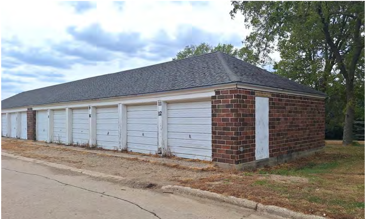
BUILDING EXTERIOR - VIEW OF NORTH EAST SIDE
