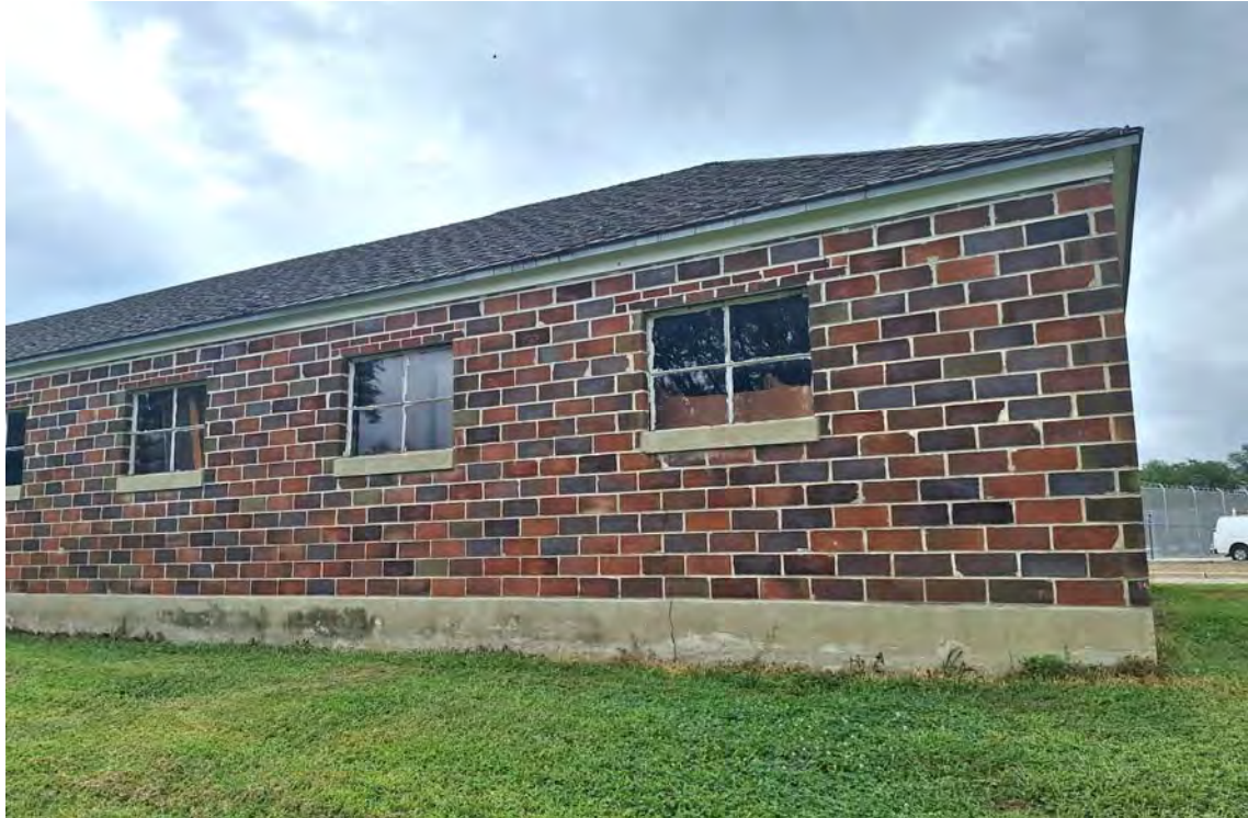
BUILDING EXTERIOR - SOUTH END OF WEST SIDE
