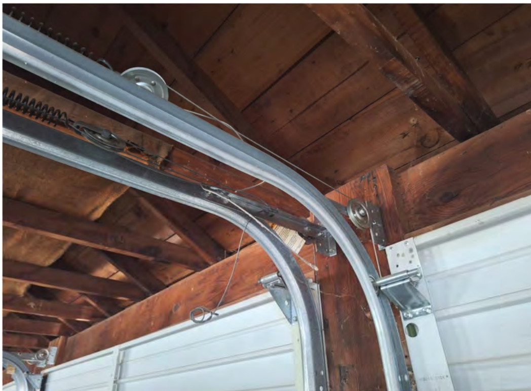
BUILDING INTERIOR - EXISTING TRACK AND SPRINGS
