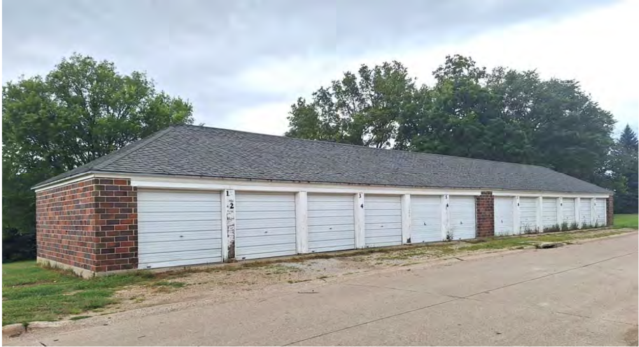
BUILDING EXTERIOR - VIEW OF EAST SIDE
