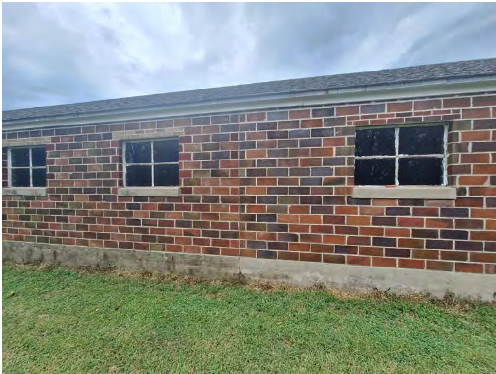
BUILDING EXTERIOR - CENTER JOINT ON WEST WALL
