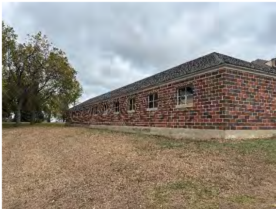
Photo #1 Overview of the CHMHI Fleet Garage west side.
