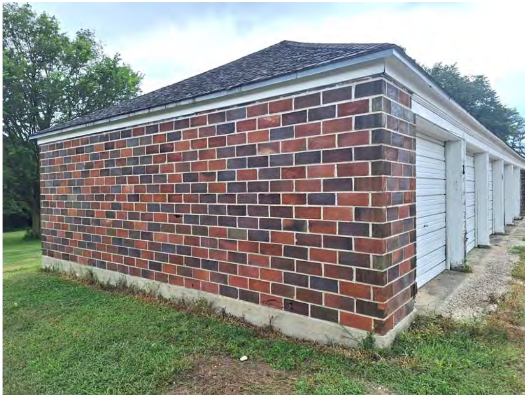
BUILDING EXTERIOR - VIEW OF SOUTH WALL
