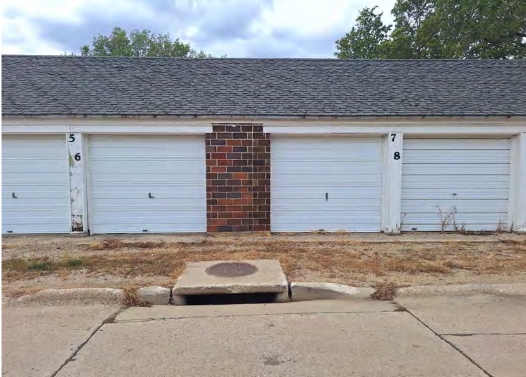
BUILDING EXTERIOR - CENTER OF EAST SIDE AT STORM INLET
