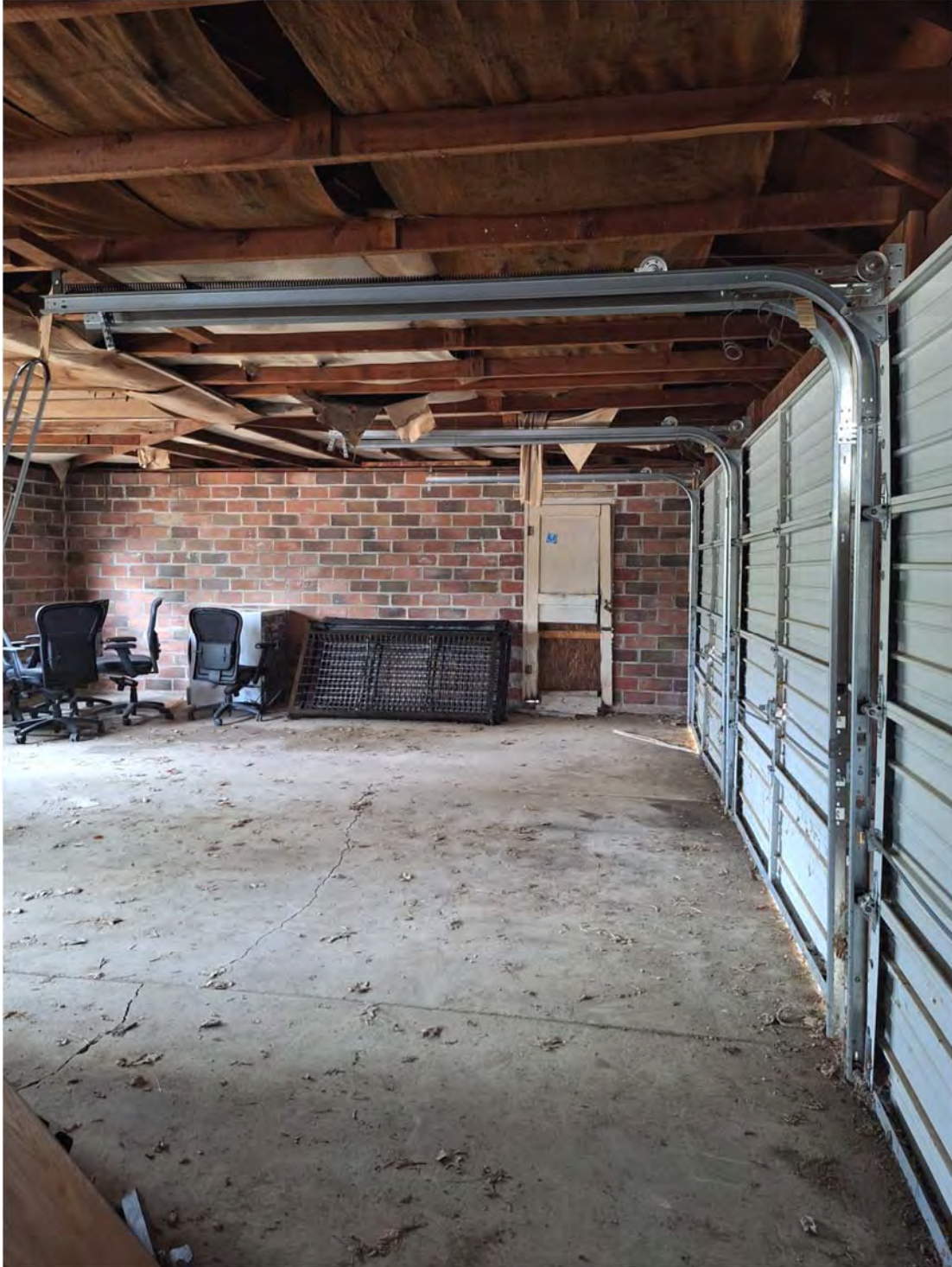
BUILDING INTERIOR - EXISTING OVERHEAD DOORS ON NORTH HALF
