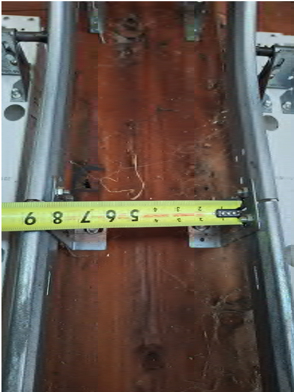
BUILDING INTERIOR - EXISTING SPACE BETWEEN TRACKS
