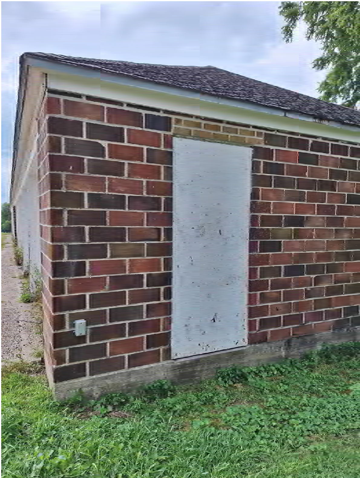
BUILDING EXTERIOR - DOOR ON NORTH END TO BE CUT WIDER
