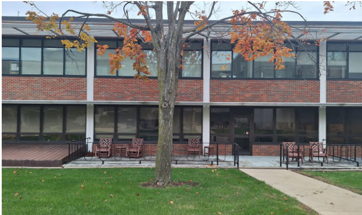
LOFTUS BUILDING - MIDDLE WEST WALL
