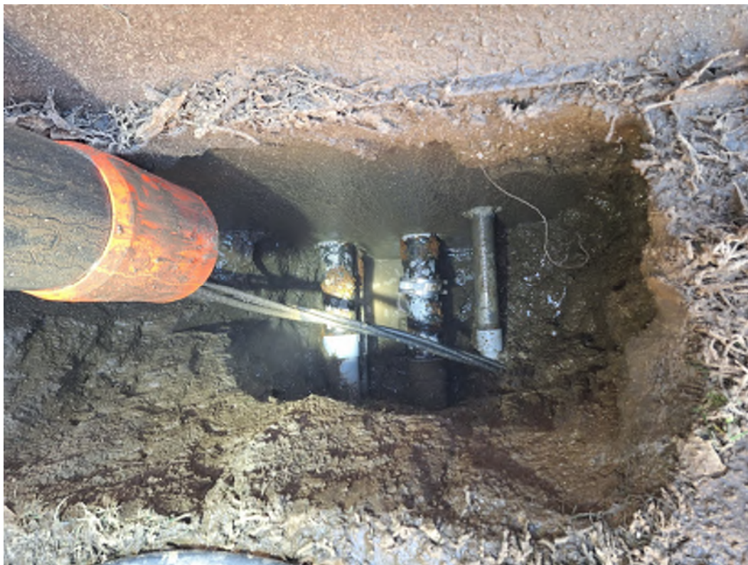
LOFTUS BUILDING - NORTH WALL - HYDROVAC AT MAIN ELECTRICAL CONDUITS
