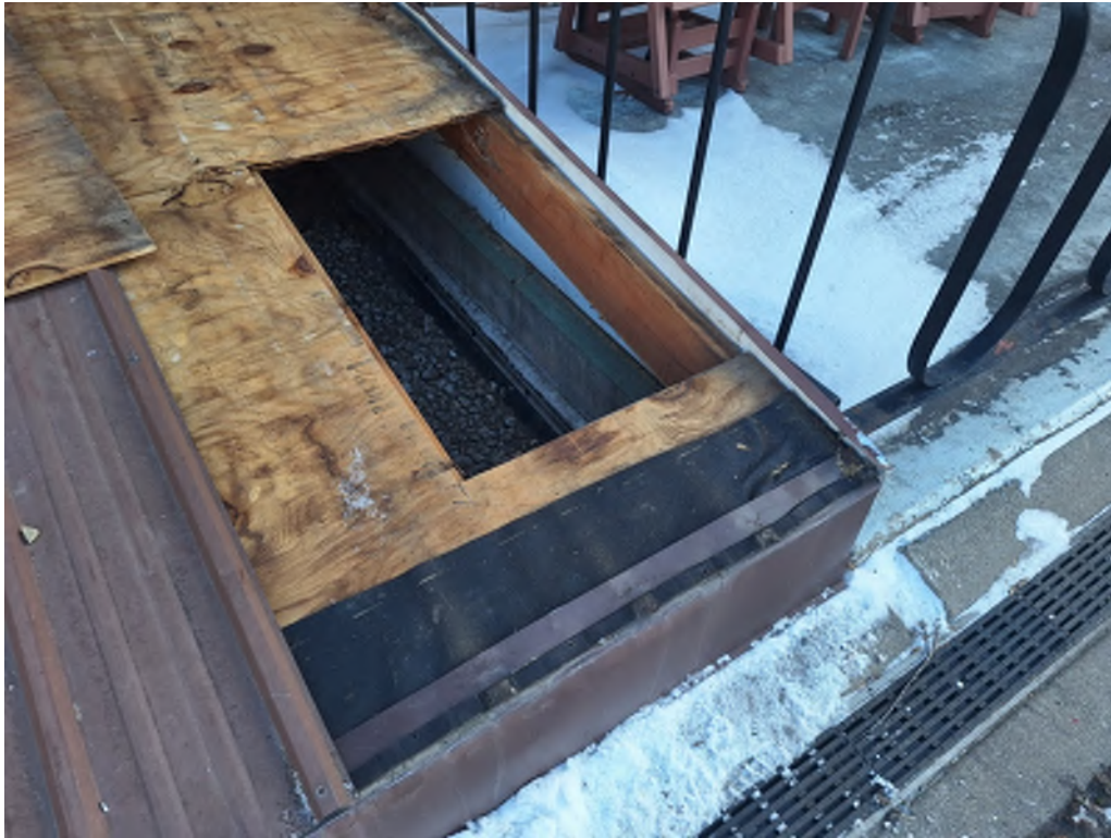
LOFTUS BUILDING - NORTH WALL - METAL ROOF EXPLORATORY DEMO
