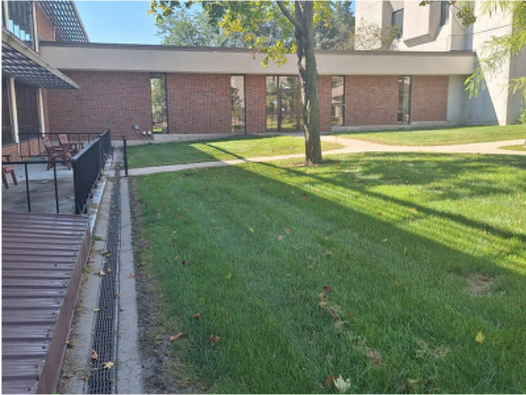
LOFTUS BUILDING - WEST WALL NORTH END - TRENCH AREA NEAR PATIO DECK
