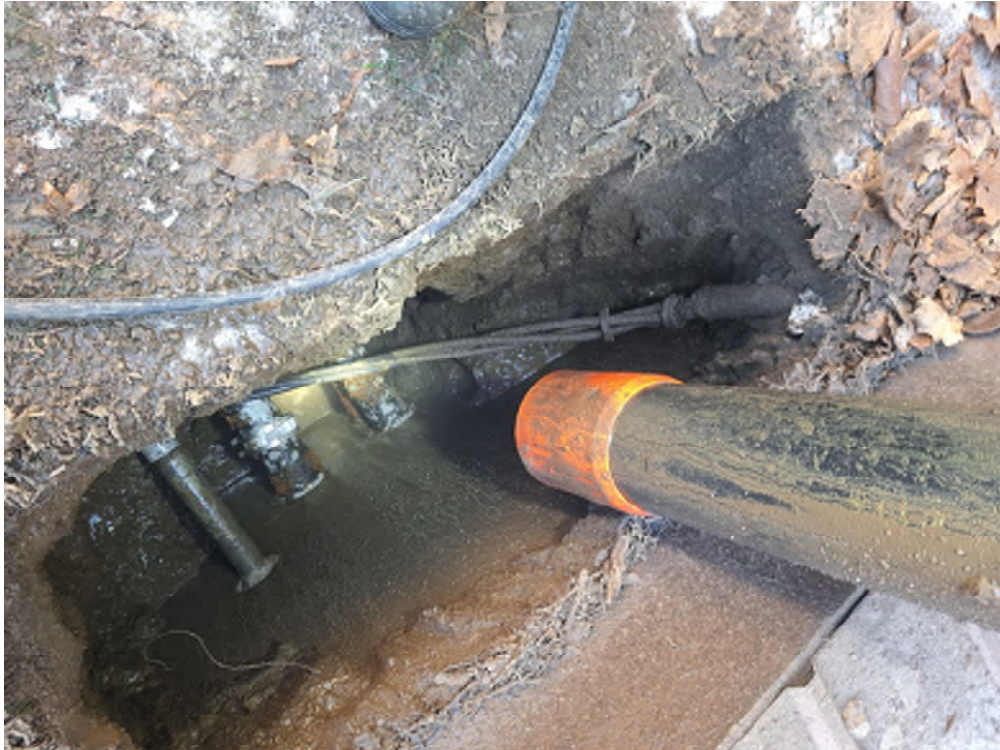
LOFTUS BUILDING - SOUTH WALL - HYDROVAC AT MAIN ELECTRICAL CONDUITS
