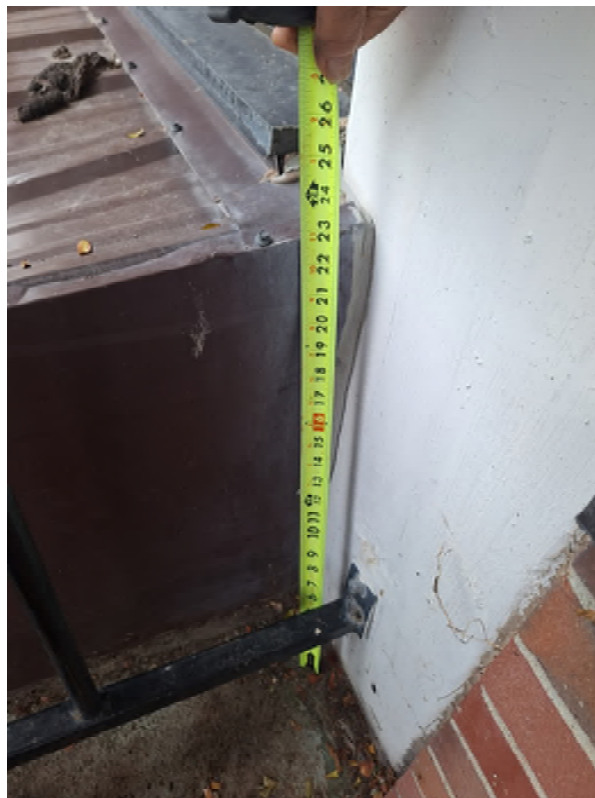
LOFTUS BUILDING - NORTH WALL - METAL ROOF BACK FLASHING TRIM
