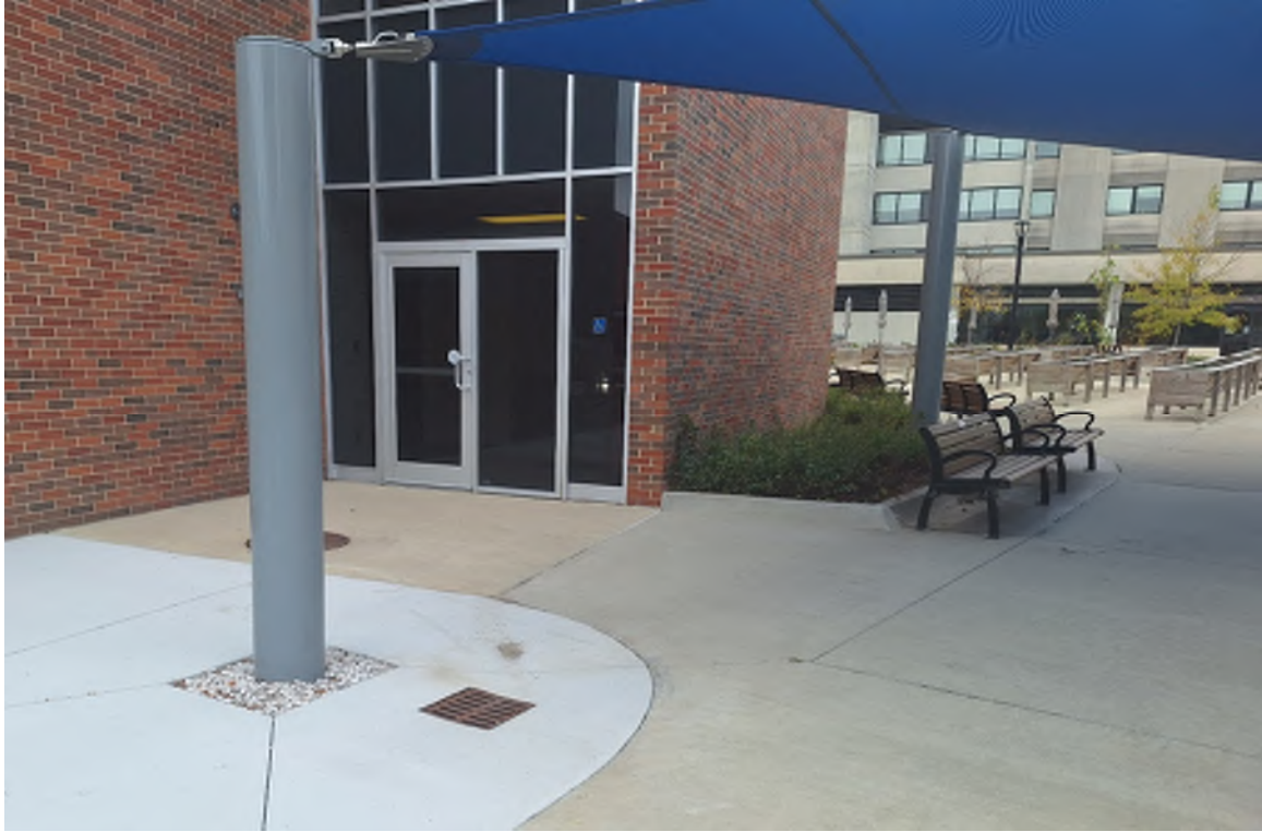
LOFTUS BUILDING - NORTH WALL - EAST SIDE - SHORING AREA AT TUNNEL
