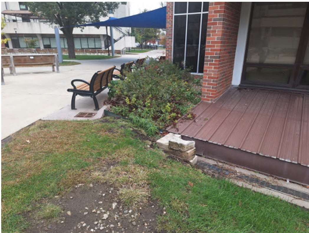
LOFTUS BUILDING - NORTH END WEST WALL - EXISTING STORM INLETS
