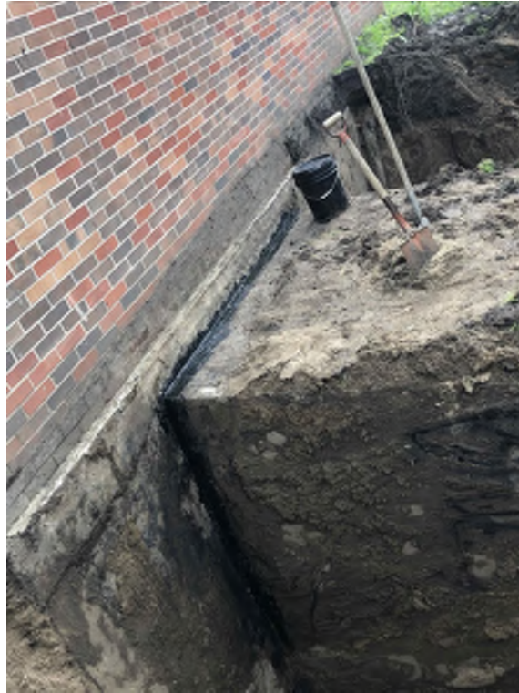
LOFTUS BUILDING - NORTH TUNNEL - PREVIOUS EXCAVATION WATERPROOFING
