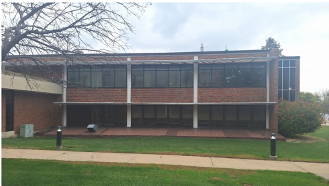
LOFTUS BUILDING - WEST WALL SOUTH HALF
