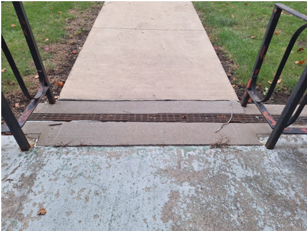
LOFTUS BUILDING - NORTH WALL - TRENCH DRAIN AND HANDRAIL WORK
