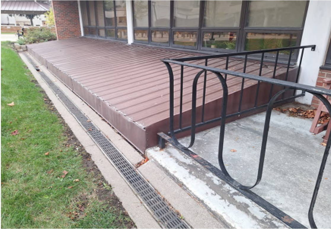
LOFTUS BUILDING - NORTH WALL - METAL ROOF AND PATIO DECK
