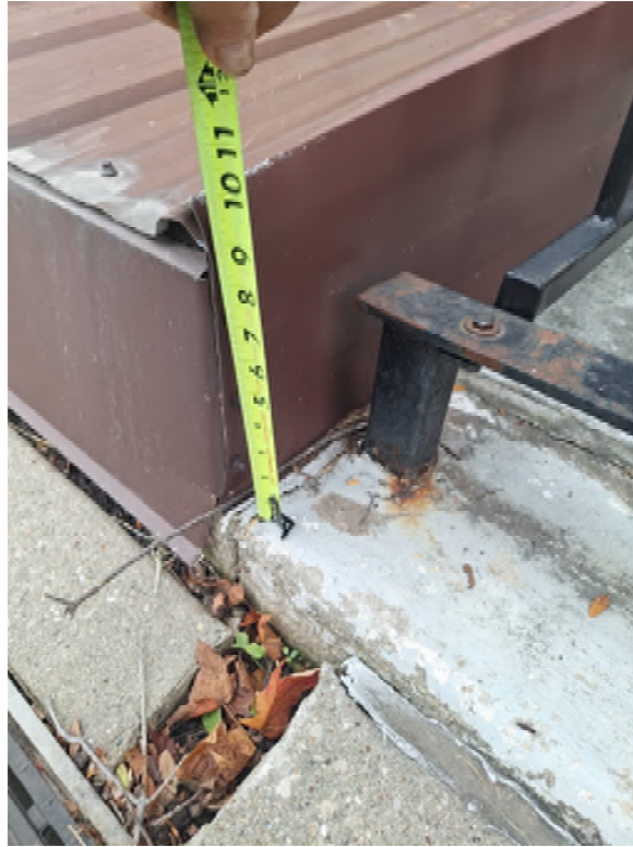
LOFTUS BUILDING - NORTH WALL - METAL ROOF FRONT FASCIA
