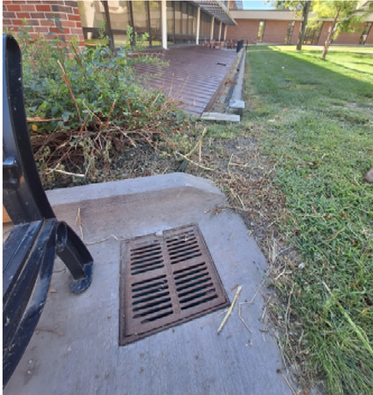
LOFTUS BUILDING - WEST WALL NORTH END OF TRENCH
