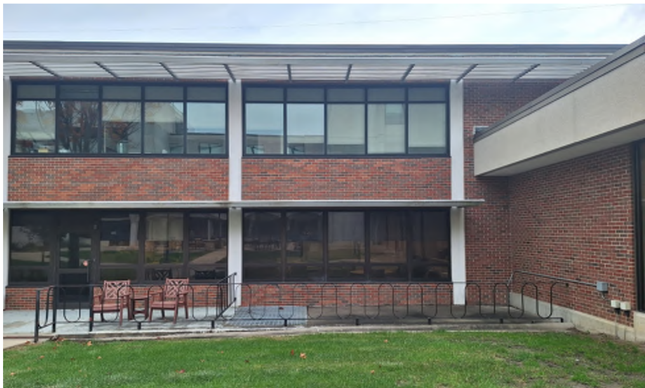
LOFTUS BUILDING - SOUTH END WEST WALL
