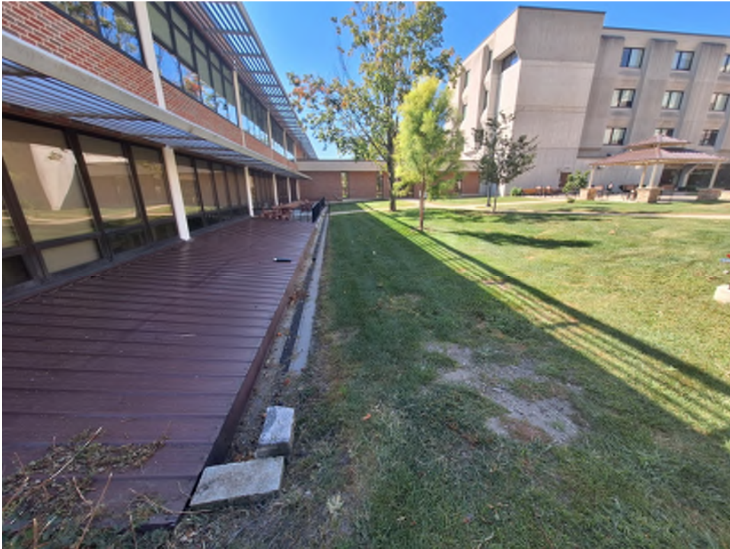
LOFTUS BUILDING - NORTH END WEST WALL - TRENCH AREA
