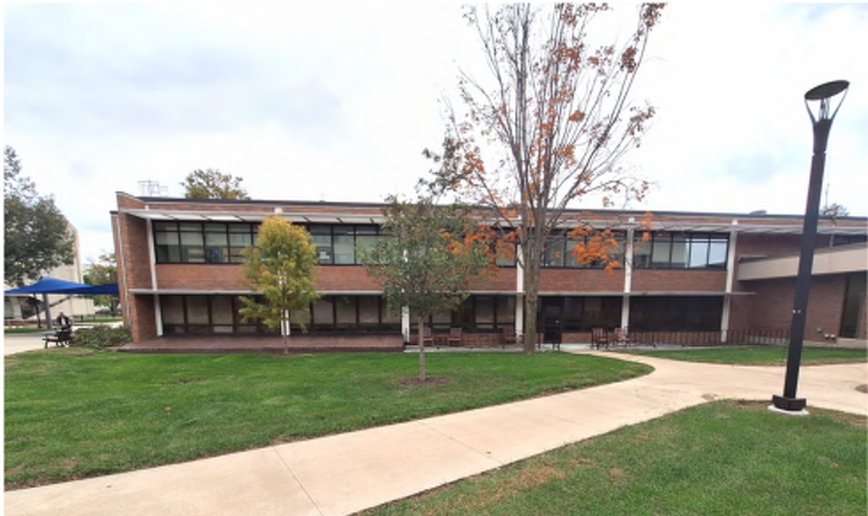
LOFTUS BUILDING - WEST WALL NORTH HALF
