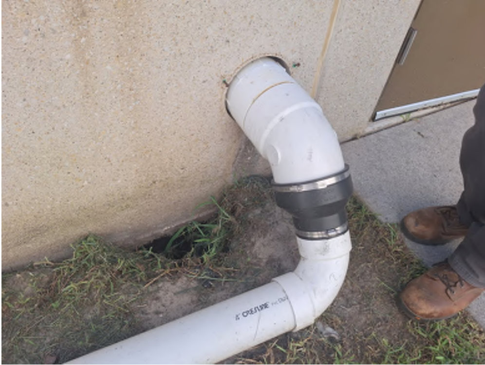
MALLOY BUILDING - NORTH KITCHEN ROOF DRAIN PIPING TO GO UNDERGROUND
