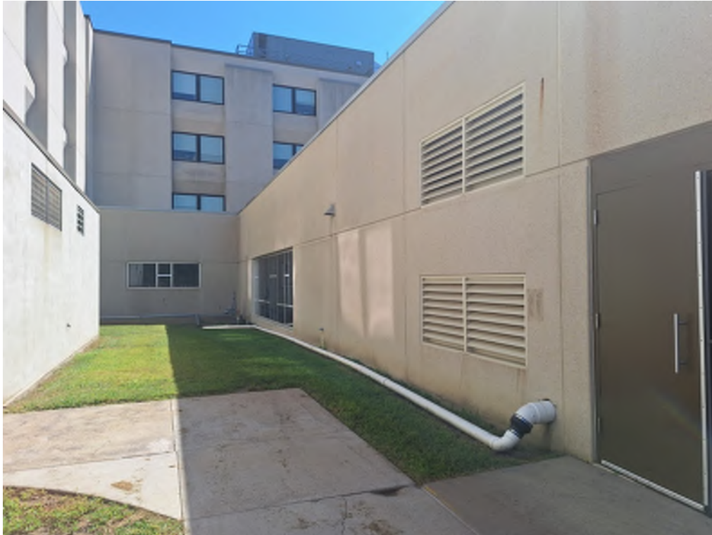
MALLOY BUILDING - NORTH KITCHEN TRENCH & ROOF DRAIN PIPING LOCATION
