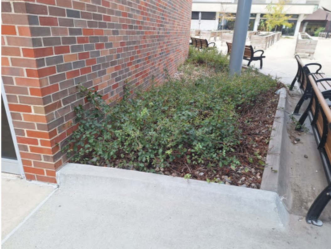
LOFTUS BUILDING - NORTH WALL - CURB DEMO AND AWNING POST AT TUNNEL
