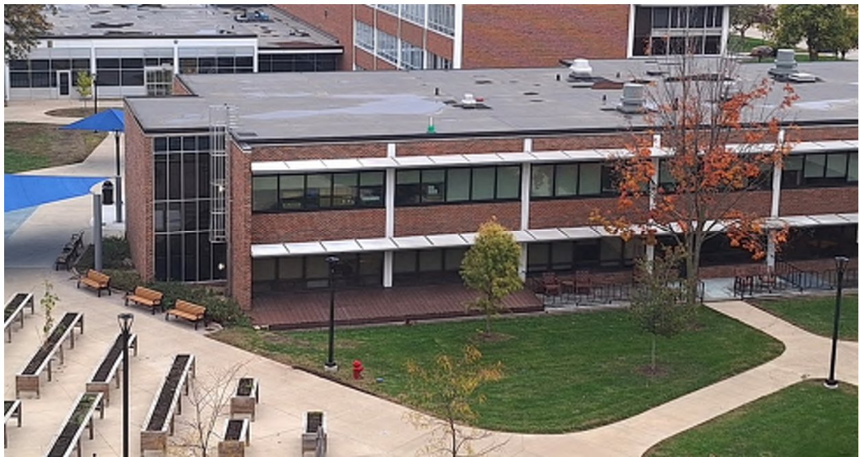
LOFTUS BUILDING - WEST WALL NORTH HALF
