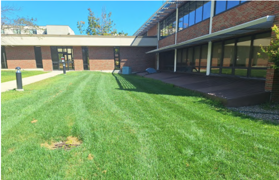
LOFTUS BUILDING - SOUTH WALL - TRENCH AREA
