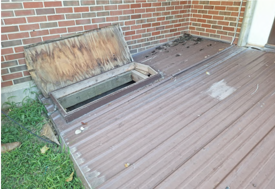
LOFTUS BUILDING - SOUTH WALL - ROOF HATCH AT NORTH END
