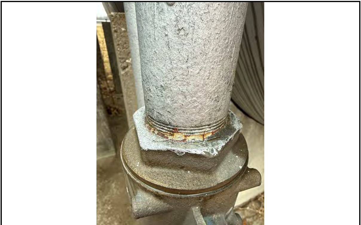
Photo 4: View of white pipe sealant
