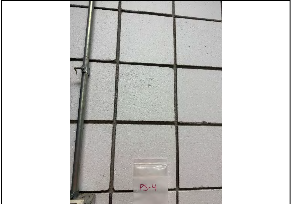
Photo 1: View of PS-4 sample location, paint is 0.0065% lead by weight
