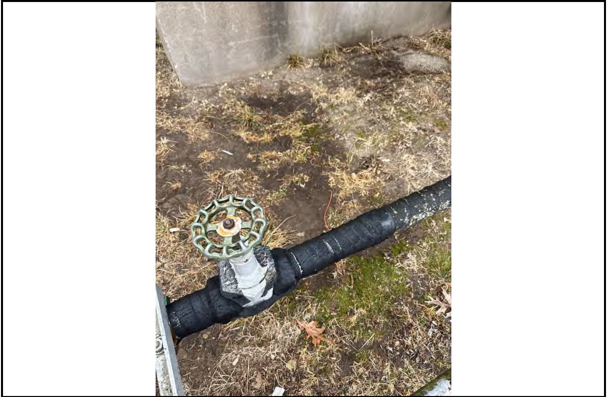
Photo 3: View of black piping wrap/insulation
