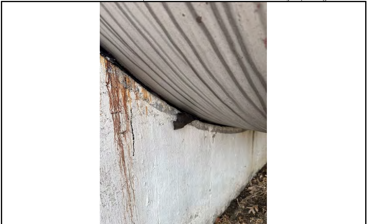
Photo 2: View of tank saddles with black tar paper/gasket
