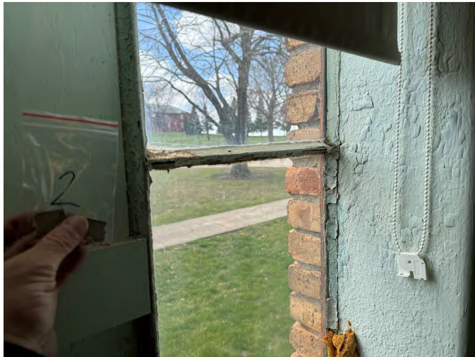
View of the ACM Window Glazing. (PP-2, 3% Chrysotile)
