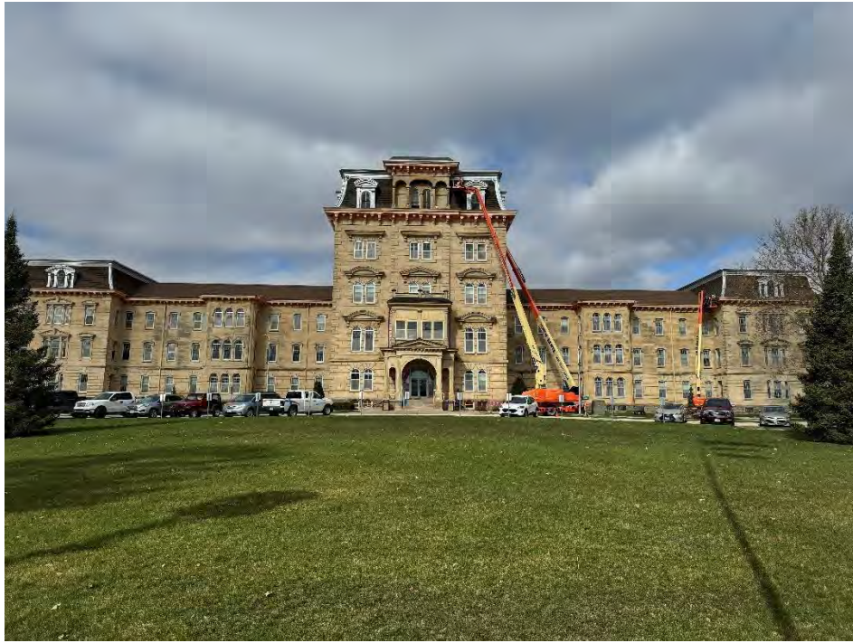
Exterior view of IMHI main entrance.
