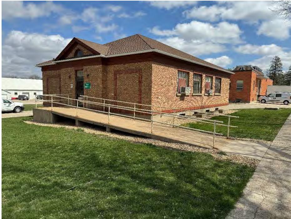
View of the Plant Operations Building.
