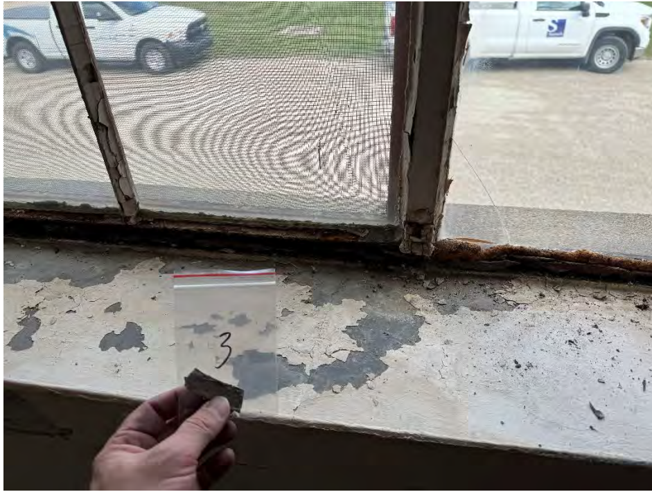
View of the ACM Window Glazing. (PP-3, 3% Chrysotile)
