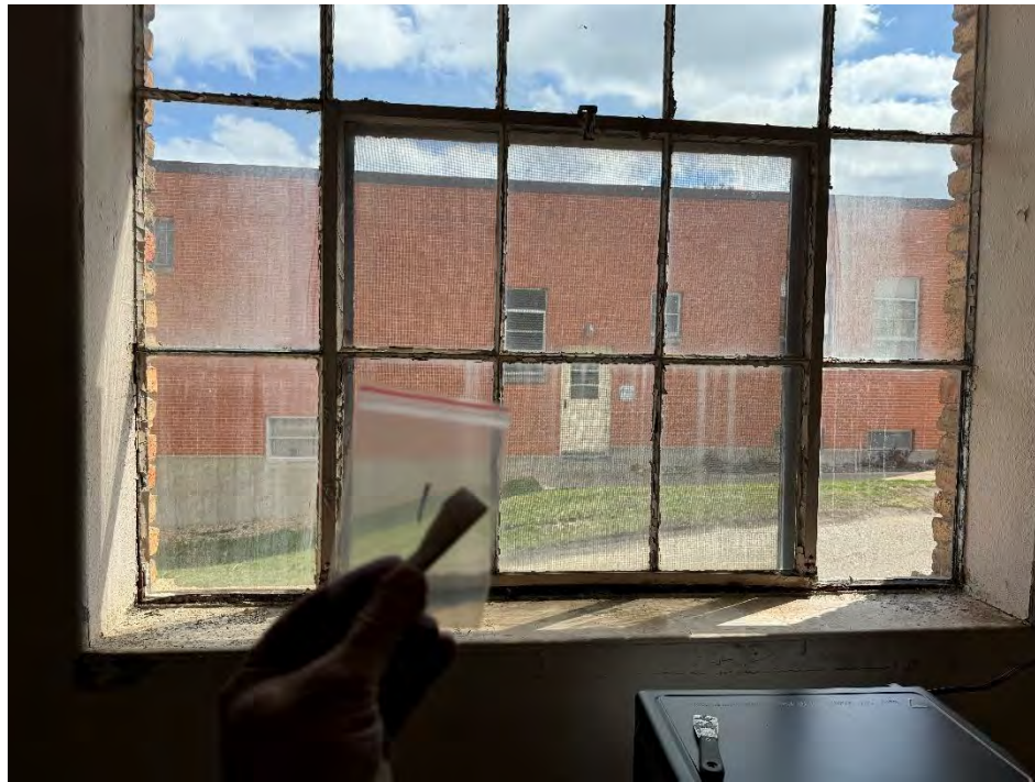
View of the ACM Window Glazing. (PP-1, 3% Chrysotile)
