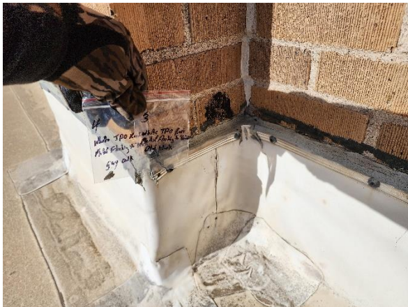
Photo #3 Sample 3. Asbestos containing black caulking/flashing on the north wall of the lower white TPO roof.
