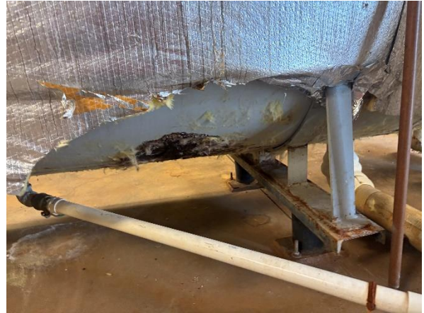
Photo #2 Building G, Underside of Water Tank, Showing base, Insulation and Grey Paint.
