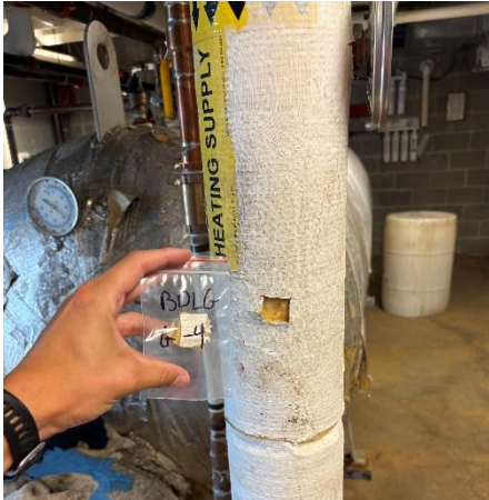
Photo #1 Bldg-G-4 Non-Asbestos Containing, Showing Heating Supply pipe and Water Tank.
