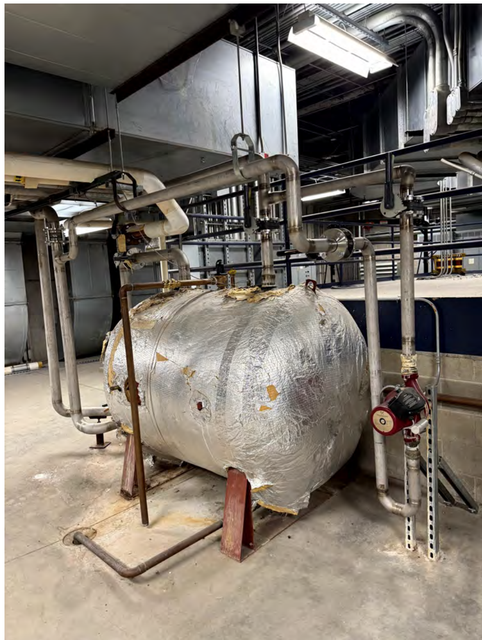
PHOTO 1 FACING NORTH EAST
