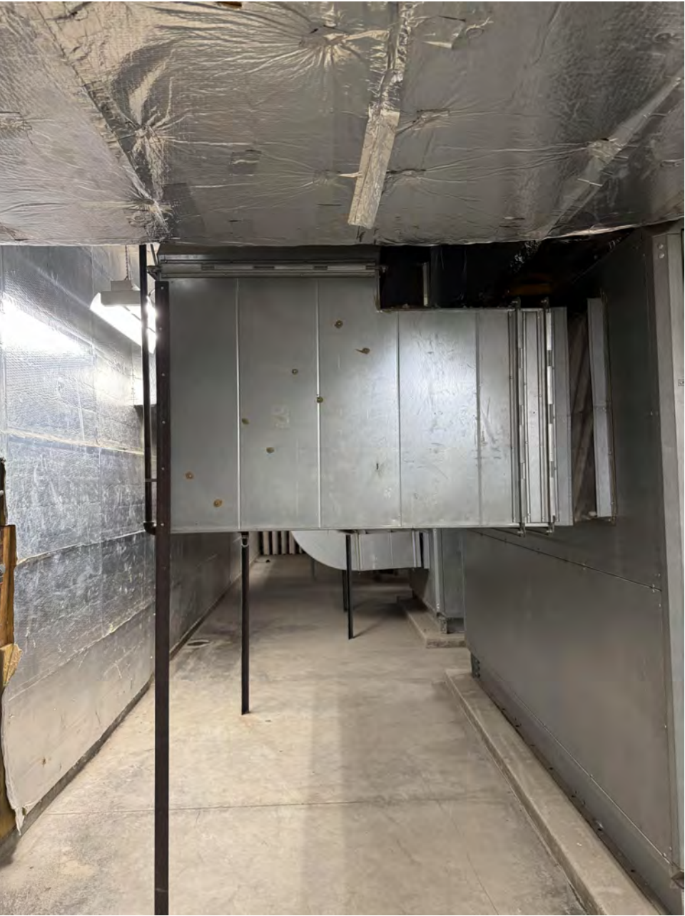
PHOTO 8 FACING WEST AT ELBOW TO REMOVED AND REINSTALLED
