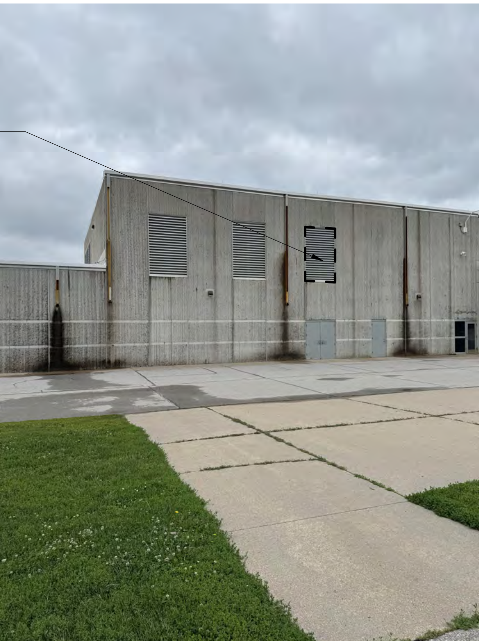
PHOTO 6 FACING NORTH AT STAGING AREA
