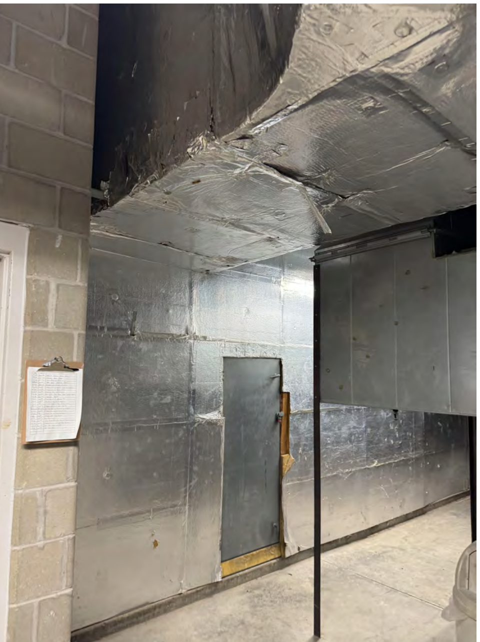
PHOTO 10 FACING SOUTH WEST AT PLENUM
