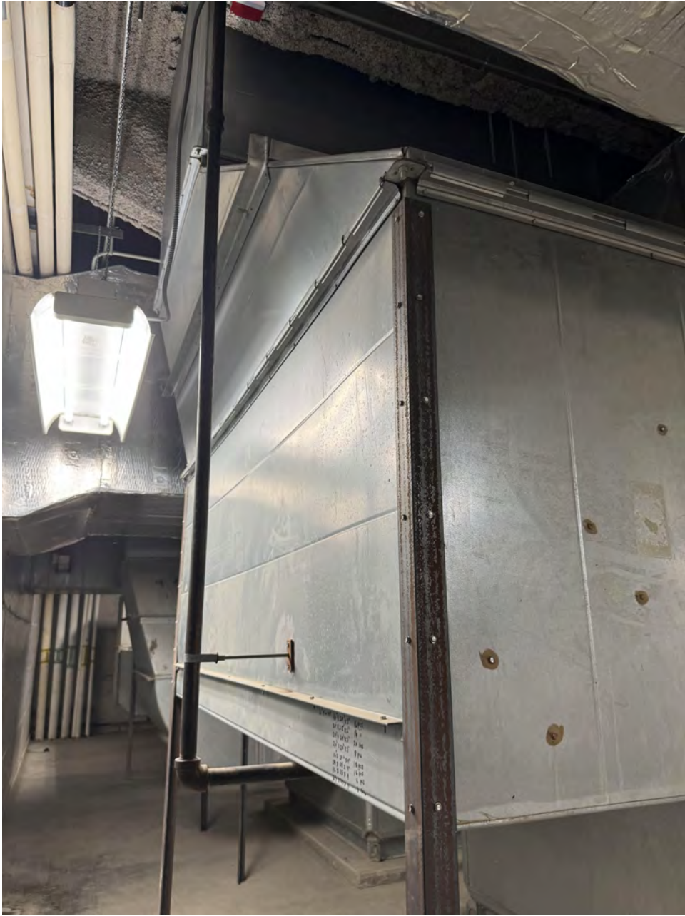
PHOTO 9 FACING WEST AT ELBOW TO REMOVED AND REINSTALLED
