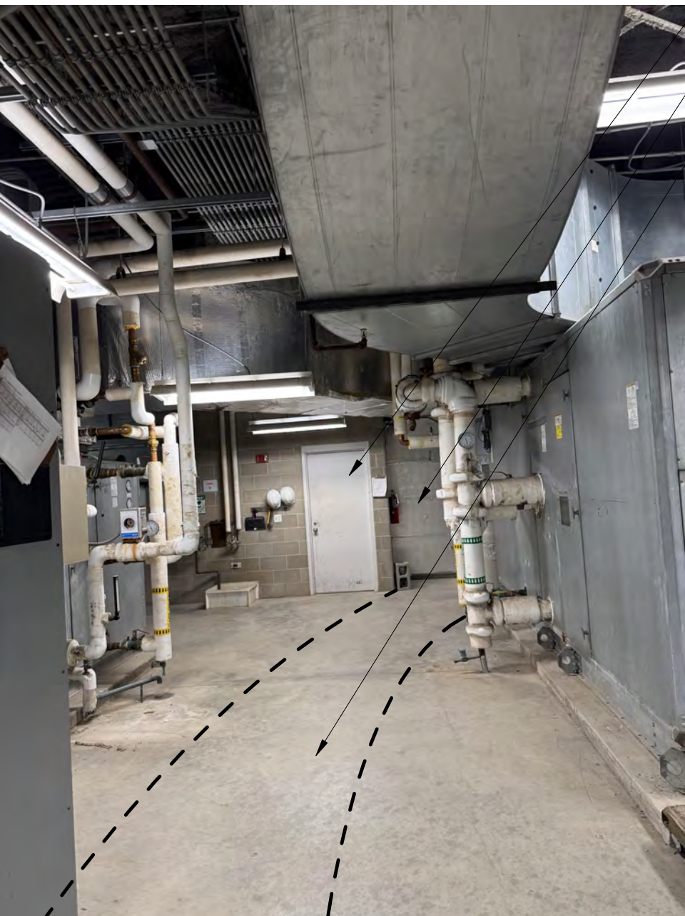
PHOTO 7 FACING SOUTH TOWARDS STAIR ACCESS AND PLENUM
