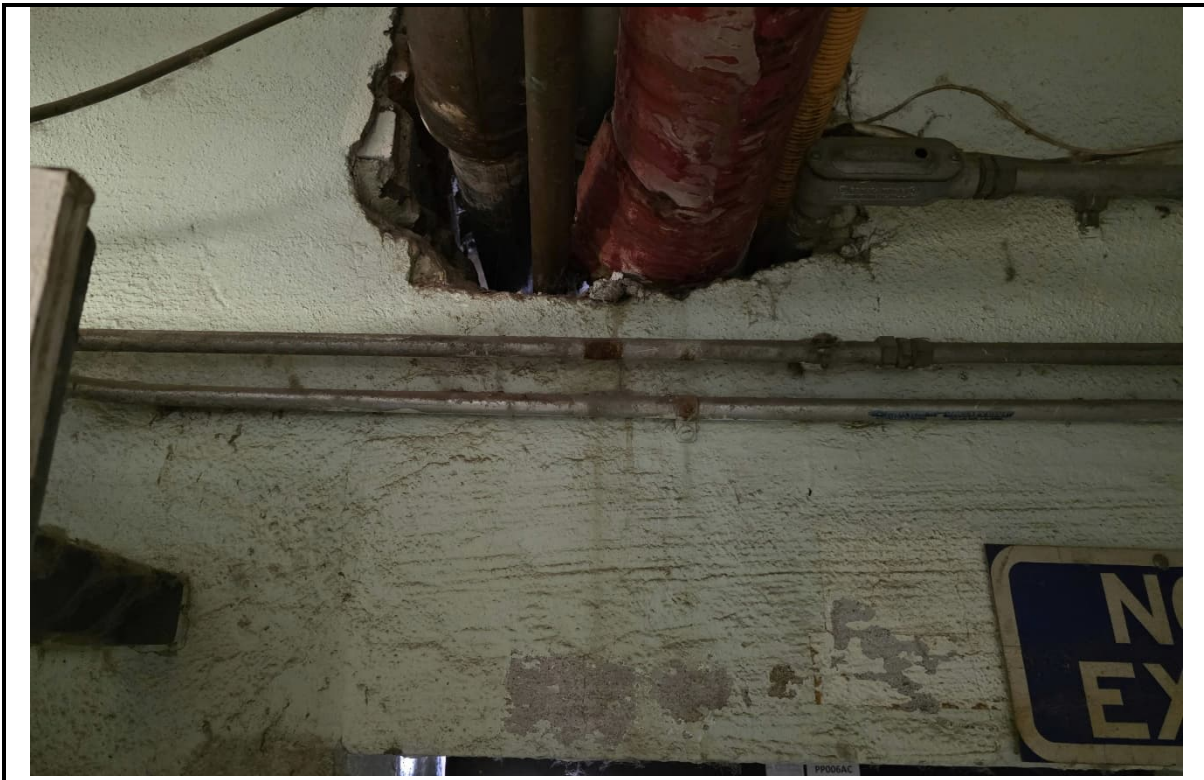
Photo 4: View of PC-2, light green lead-containing paint, located on the north Powerhouse walls.
