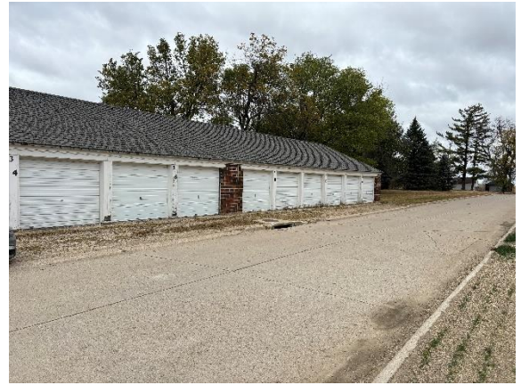
Photo #2 Overview of the CHMHI Fleet Garage east side.
