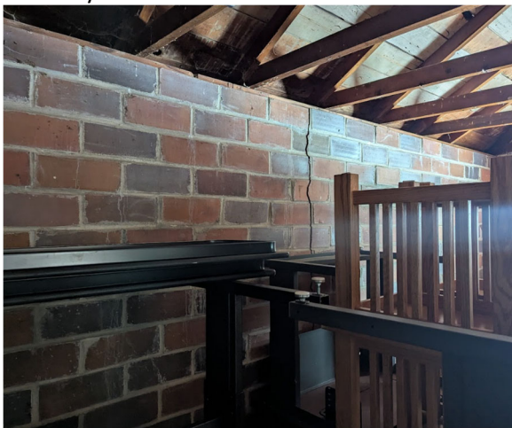
Masonry Crack on South Wall
