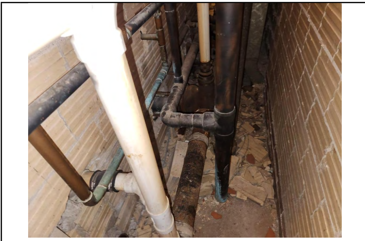
Photo 16: View of a typical pipe chase closet with cast iron, copper, and PVC piping (no ACM present).
