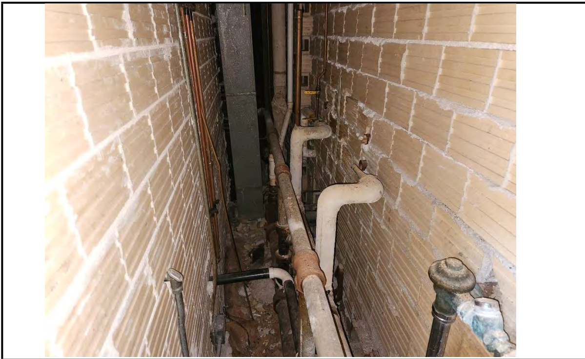
Photo 2: View of mudded joint fittings in a pipe chase in Basement Area B.
