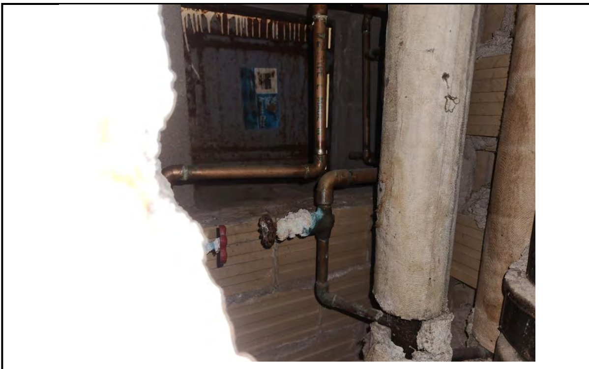
Photo 3: View of a run of vertical ACM pipe insulation.
