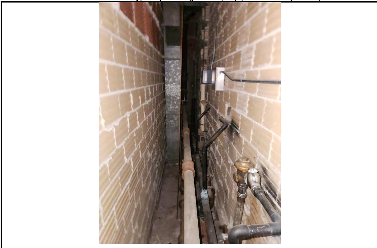
Photo 6: View of a plumbing pipe chase (no pipe insulation present).
