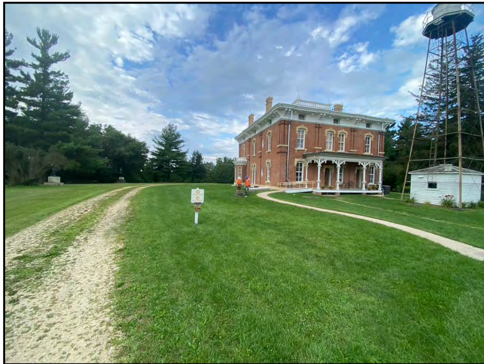
Figure 9. View of the Front Yard and East Yard, facing west.
