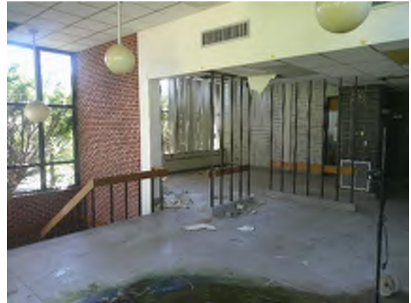
Photo #2 Overview of interior 2 nd Floor lobby of Cooper Building.
