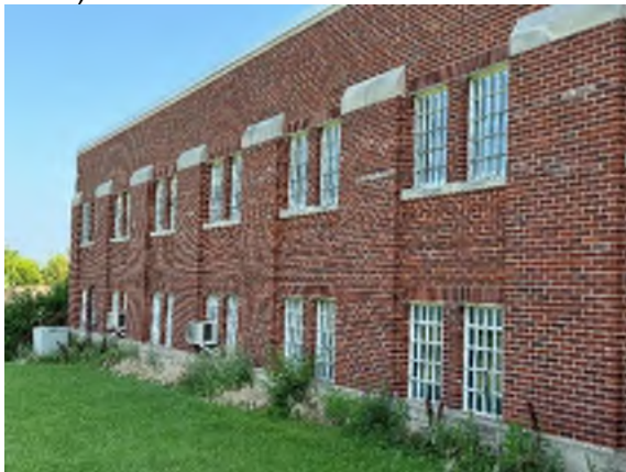
Photo #9 Overview of building exterior.
