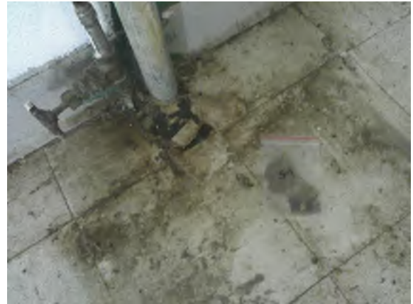
Photo #2 Asbestos containing floor tile (White w/ Gray Streaks) – 2 nd Floor Room #3 (2% Chrysotile)
