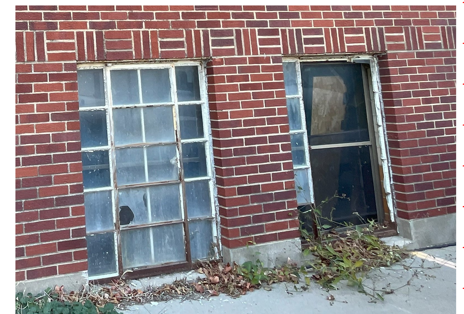
G4) TYPICAL EXISTING WINDOW CONDITION NOT TO SCALE
