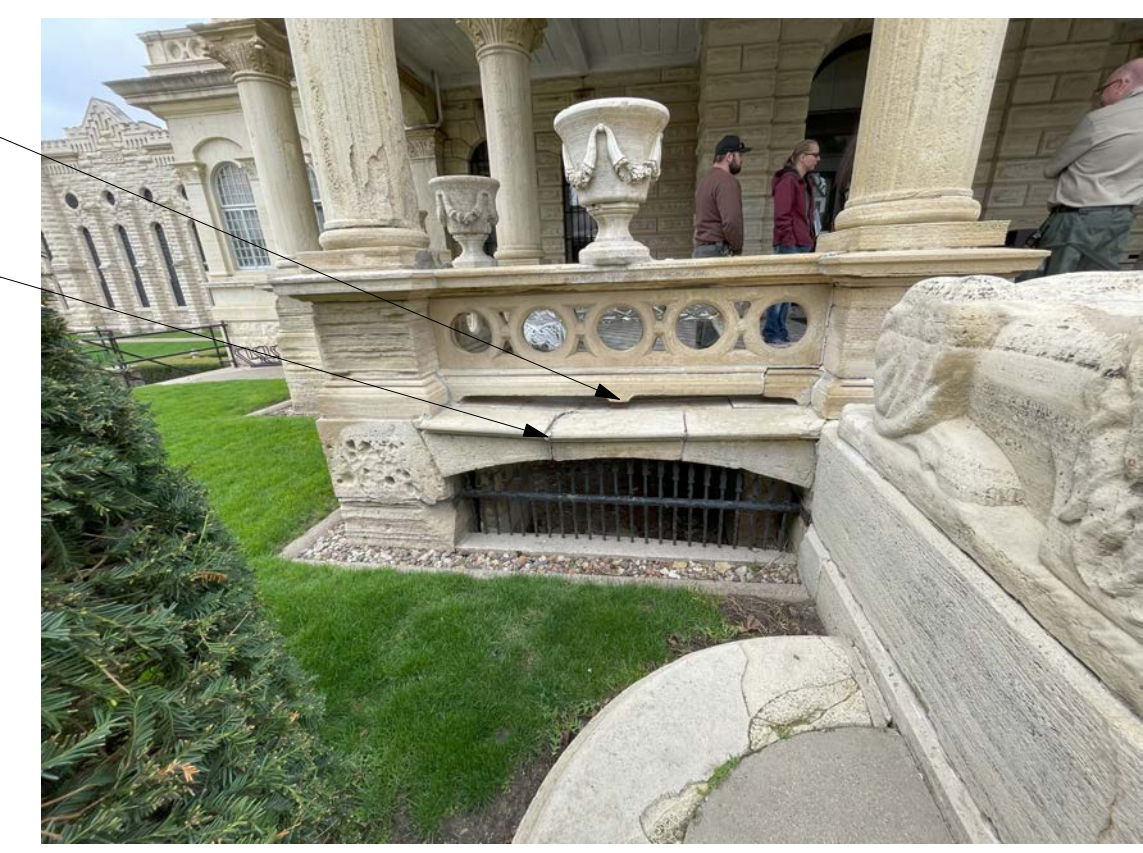
F17 PHOTOGRAPH OF STONE ARCH IN DETAIL J14/A301
