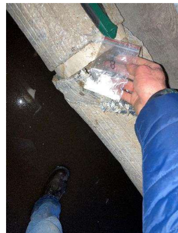
Photo #6 Asbestos: Sample #8 – 6"-8" O.D Straight Pipe Insulation Section #2 Pipe E.
