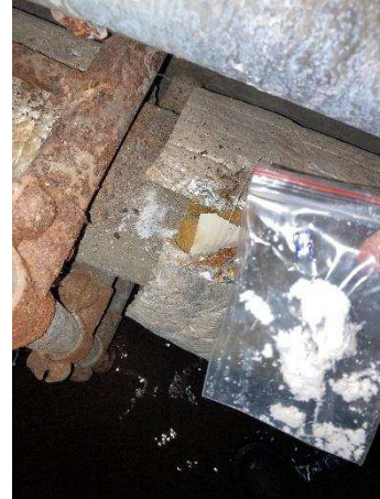
Photo #8 Asbestos: Sample #11 – 6"-8" O.D Straight Pipe Insulation Section #3 Pipe E
