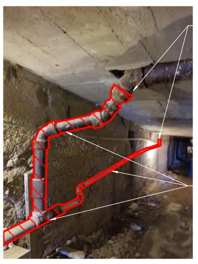
**ROUTE NEW 4" SANITARY LINE** IN TUNNEL FROM UNDERGROUND CLEAN OUT TO REMAINING 6" SANITARY PIPE THROUGH TUNNEL ROOF AND **RECONNECT. ROUTE 2"** SANITARY LINE TO EXISTING 2" PIPE THROUGH TUNNEL ROOF AND RECONNECT.
