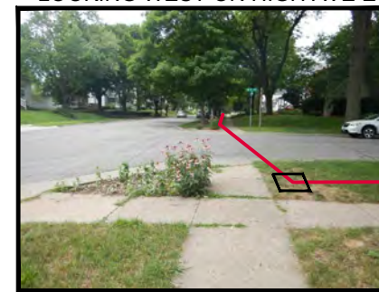
BORE PIT LOCATION ICN STA. 25+65
