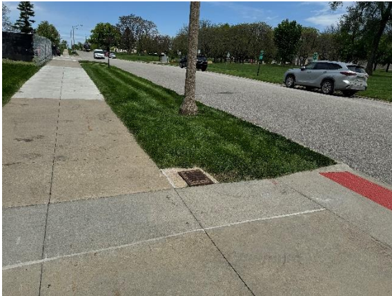
Photo #1 Looking north along E 13 th street at one of the vents.
