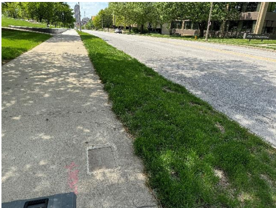
Photo #3 Looking west along E Grand Ave at one of the vents.
