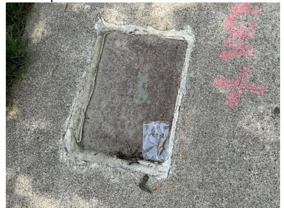
Photo #4 Caulking on metal lid at on E Grand Ave (vent 24+67 on map) Sample CCT-2
