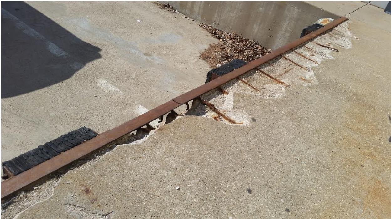
Middle of dock, facing South. Shows where concrete has eroded. 05/05/2017
