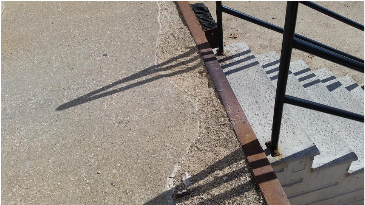
Dock area directly in front of double door entrance to building. Precast Stair (pre-failure) visible. Area where concrete eroded and filled with sand temporarily. 05/05/2017
