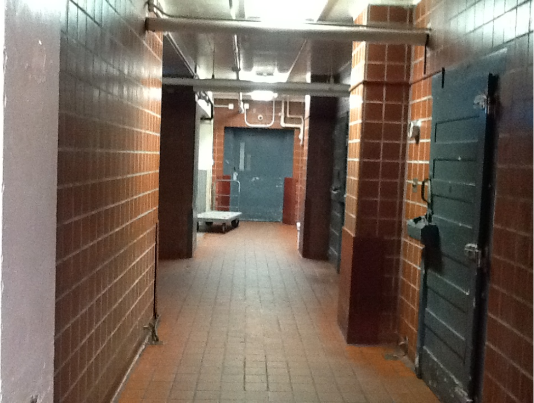
Figure 1: Remote corridor with century-old cooler unit
