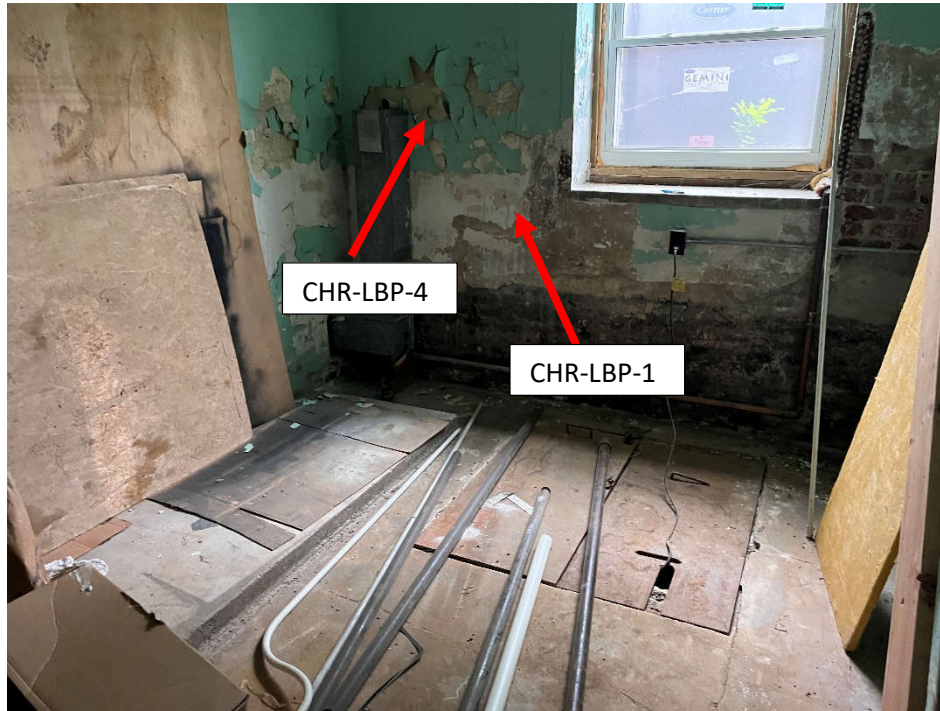
View of White and Neon Green Lead Based Paint (Samples CHR-LBP-1, 98,000 ppm and CHR-LBP-4, 190,000 ppm)
