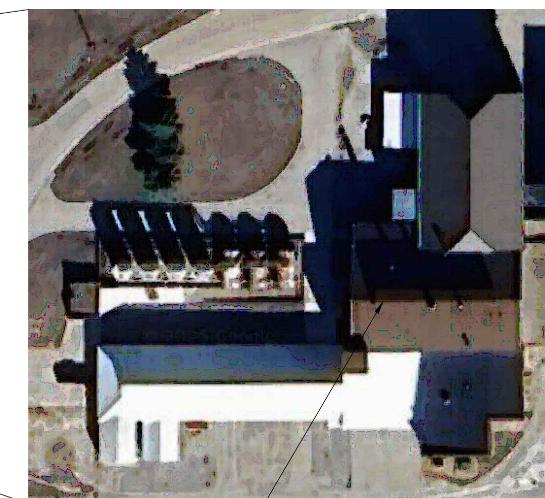
"POWER HOUSE" BOILER ROOM
