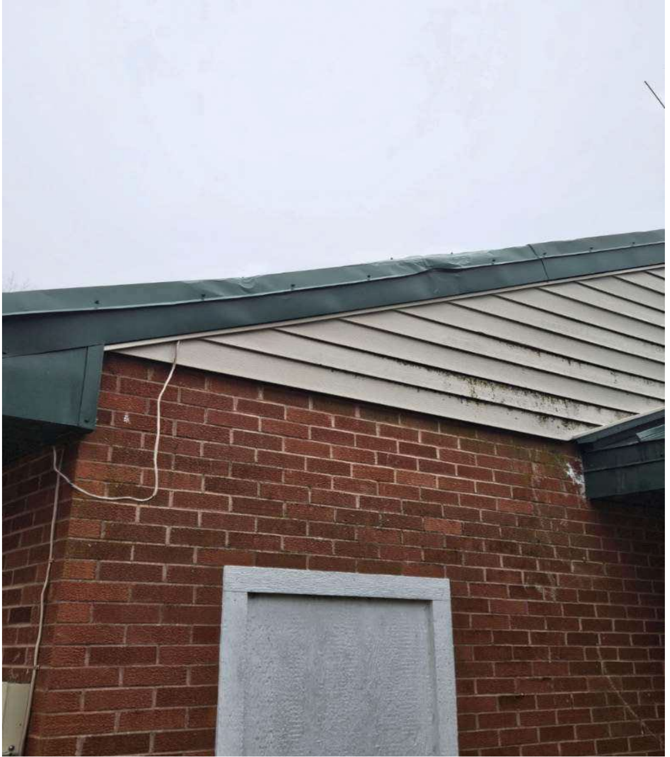
Photo 6. Existing Steel Roof Edging
