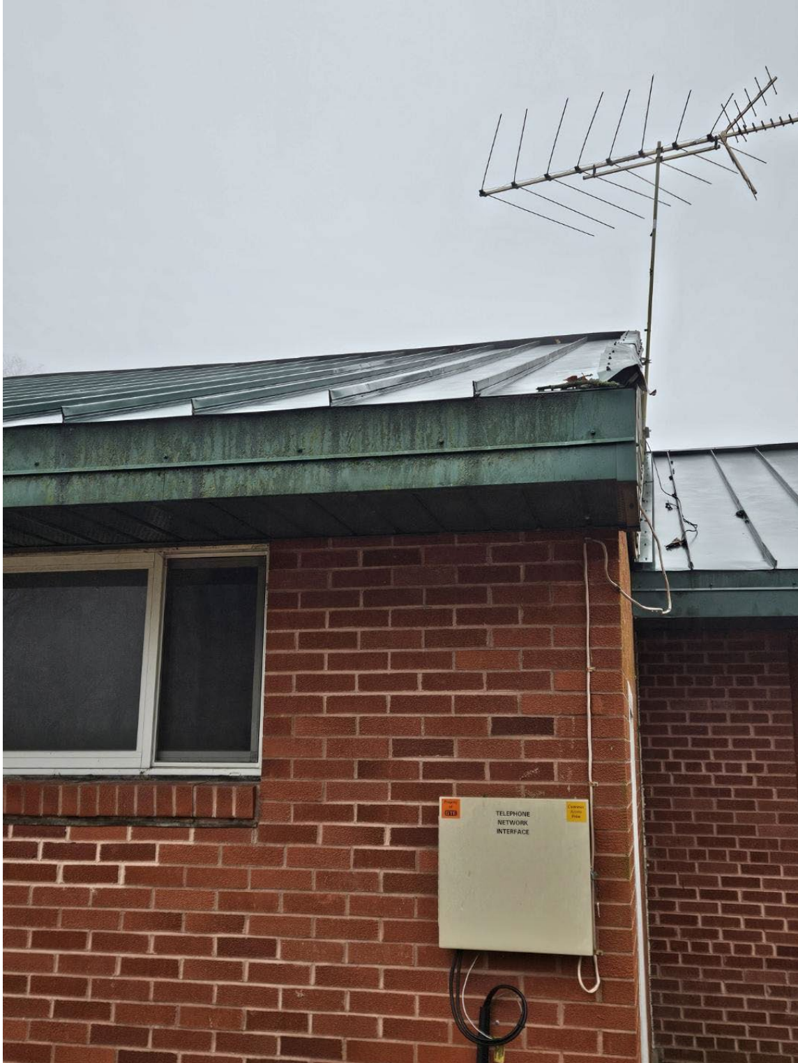
Photo 4. Existing Standing Seam Steel Roof, Steel Fascia and Steel Edge Trim
