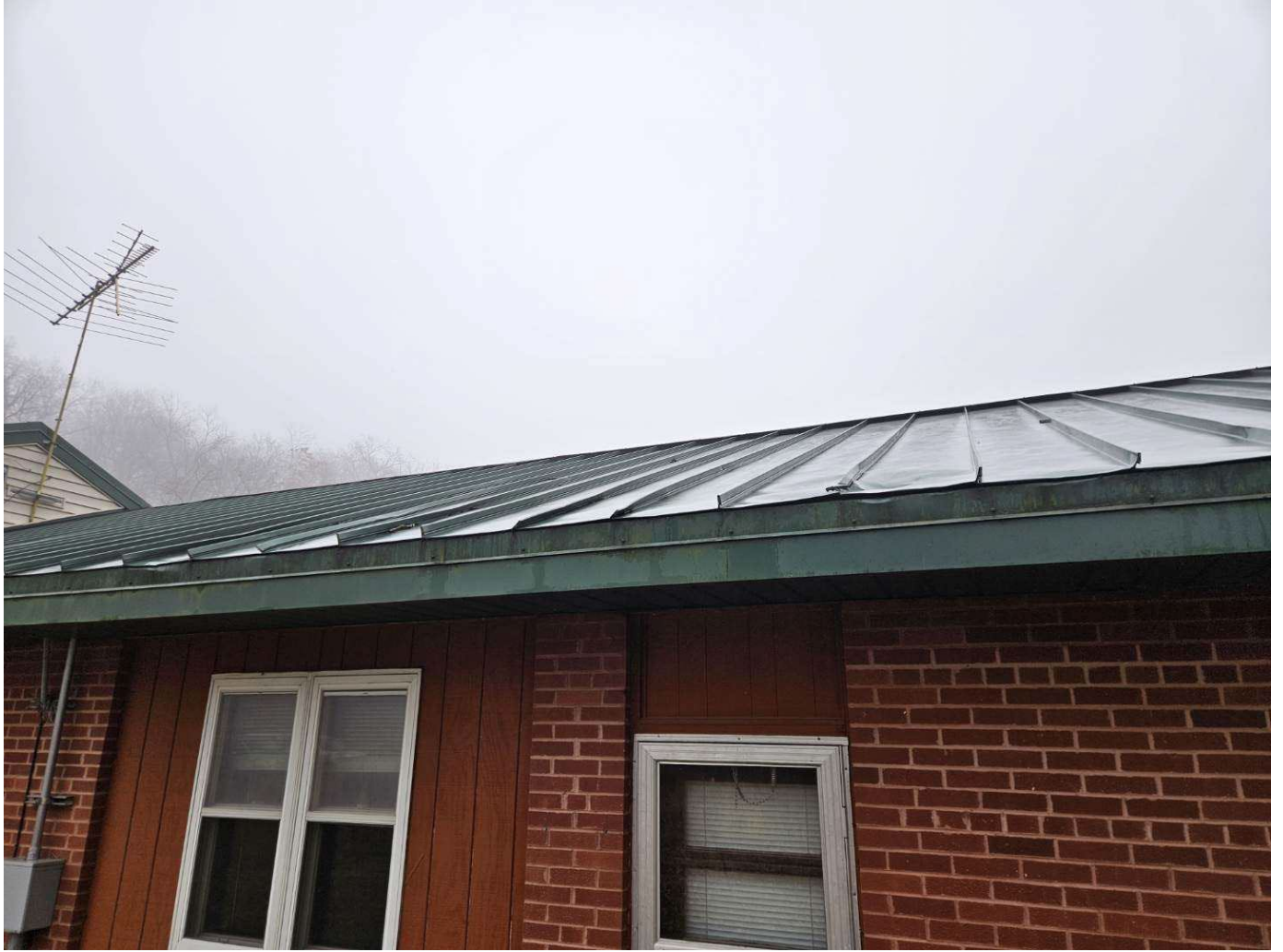
Photo 5. Existing Standing Seam Steel Roof and Steel Facia
