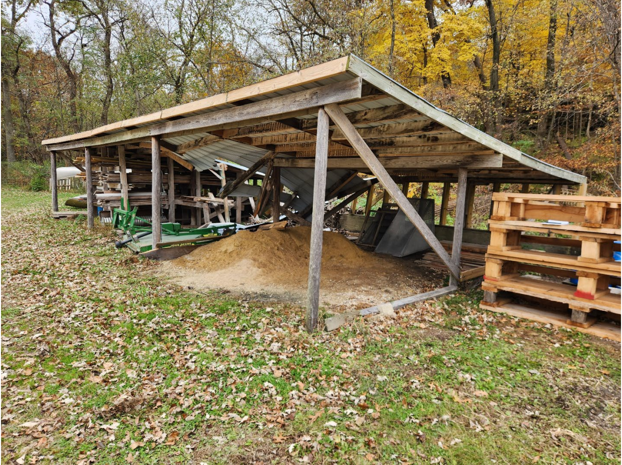
Photo 1. Existing Pole Building
