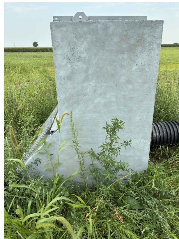
Intake Structure - Side View
