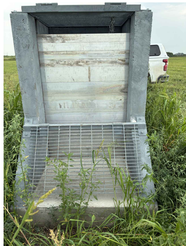
Intake Structure - Front View
