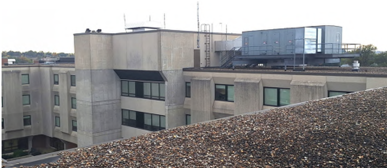
MALLOY ROOF - PENTHOUSE & LARGE RTU
