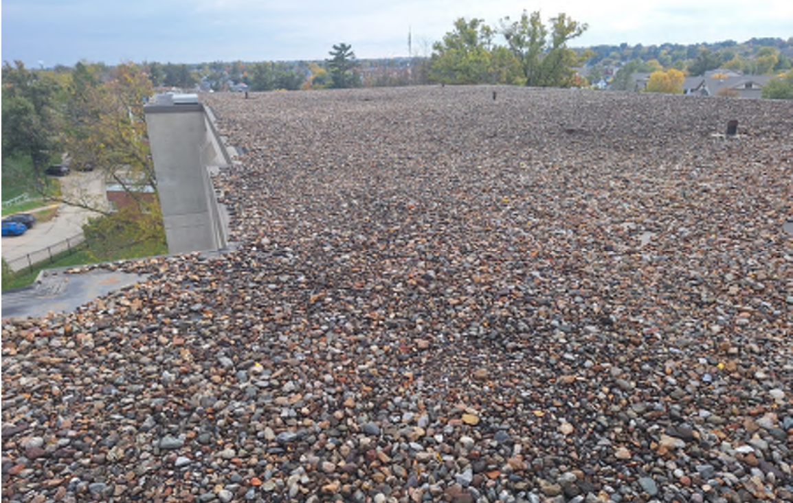
DACK ROOF - SOUTH WING
