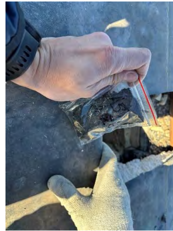
Photo #2 Sample A-6 Black Roof Tar, Dack Building ( 15% Chrysotile )
