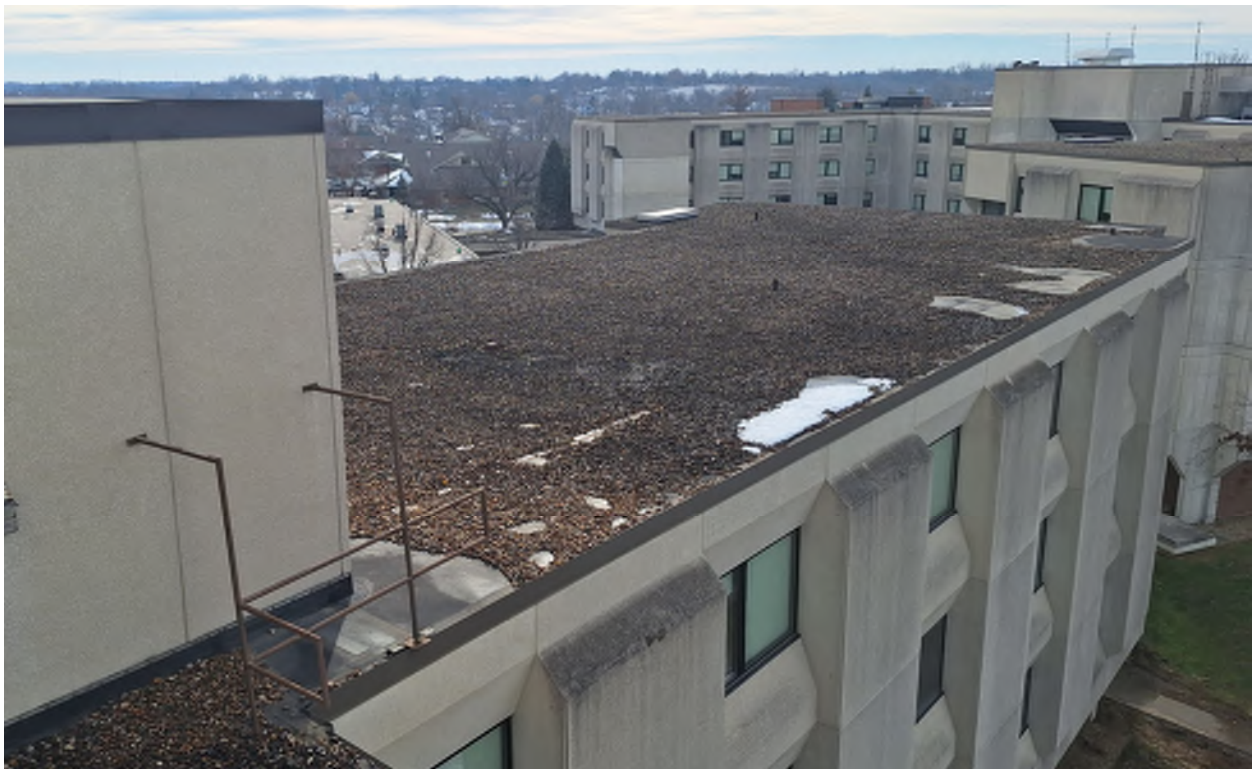
DACK ROOF - WEST WING
