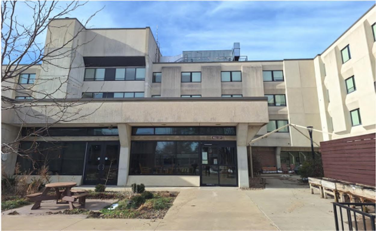
MALLOY REC CENTER NE CORNER - OVERFLOW DISCHARGE TO BE LEFT OF DOORS
