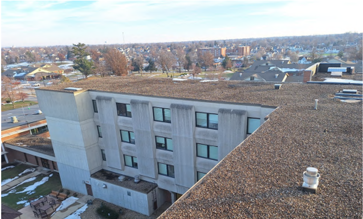
MALLOY ROOF - SOUTHEAST WING & LOWER ROOF
