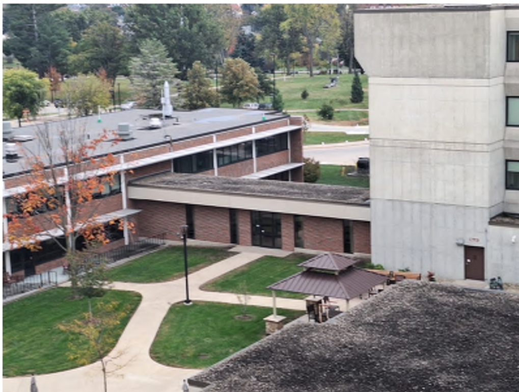
LOFTUS-MALLOY CONNECTING CORRIDOR ON COURTYARD SIDE
