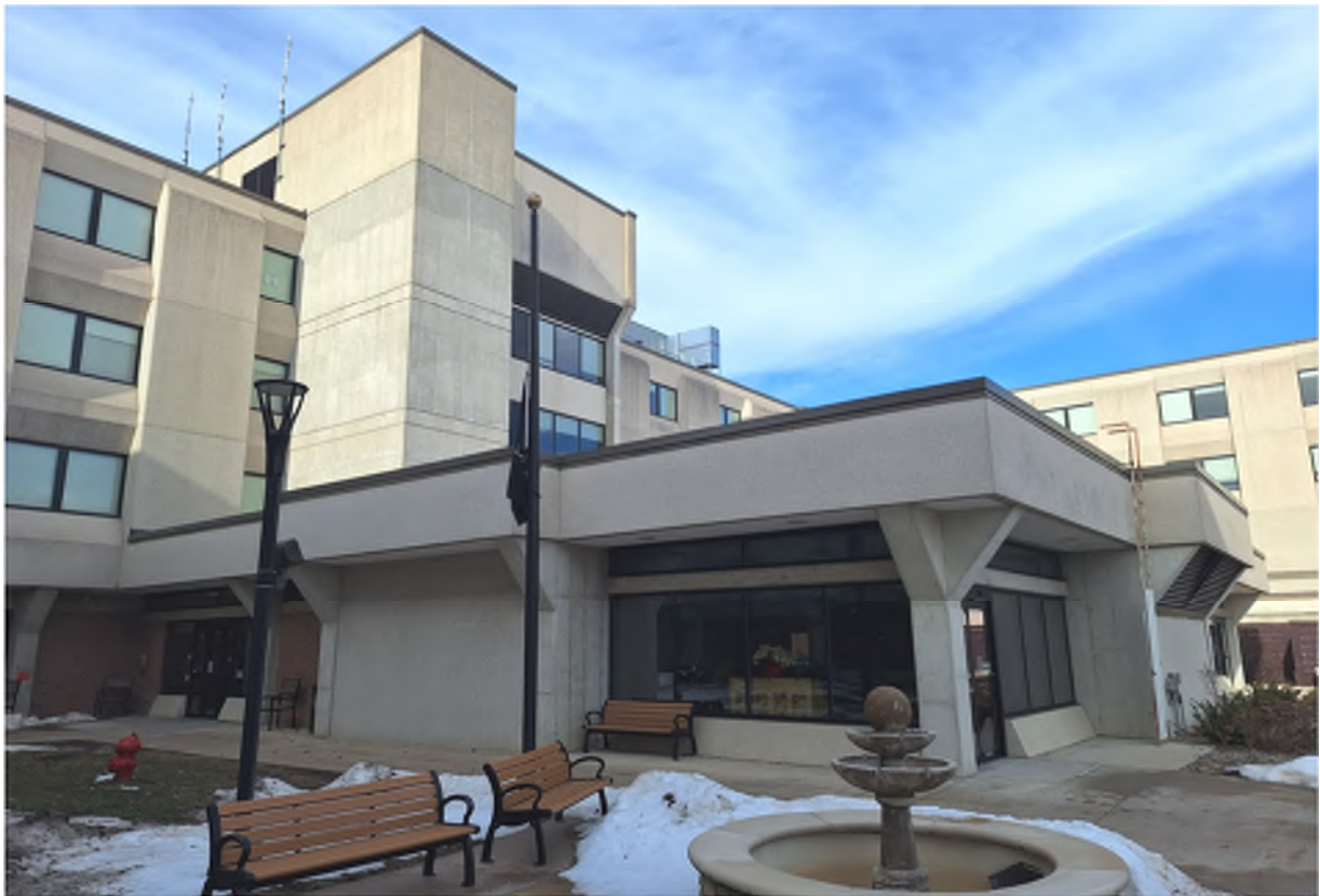
MALLOY REC CENTER - SE CORNER W/ LADDER ON RIGHT
