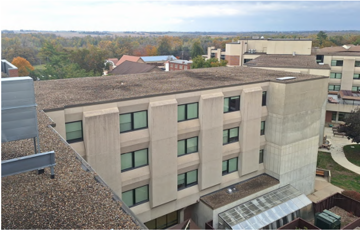
MALLOY ROOF - NORTHEAST WING & LOWER ROOF
