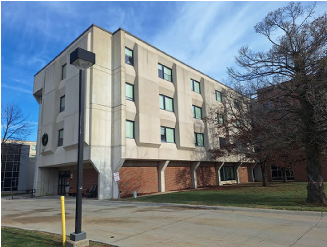
MALLOY BUILDING EXTERIOR - SOUTHWEST ROOF ACCESS AREA
