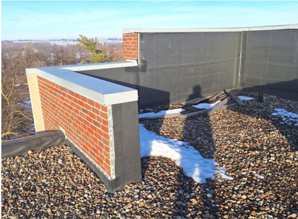
MALLOY ROOF - NORTH ENTRANCE ADDITION PARAPET WALLS
