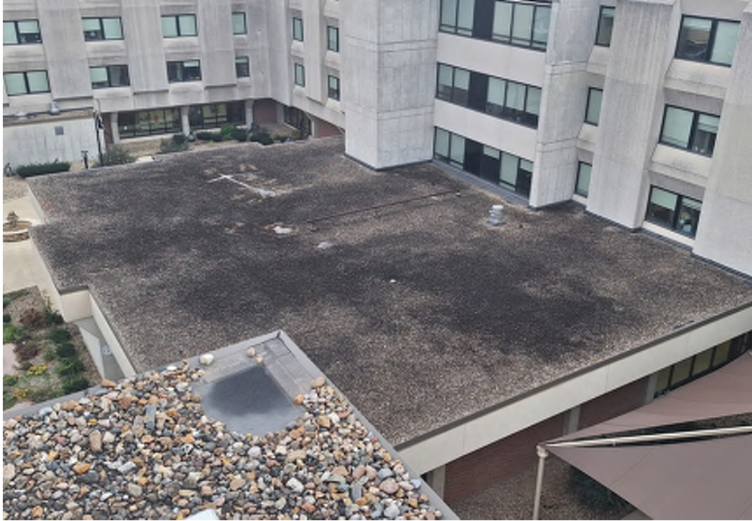
MALLOY ROOF - REC CENTER ROOF
