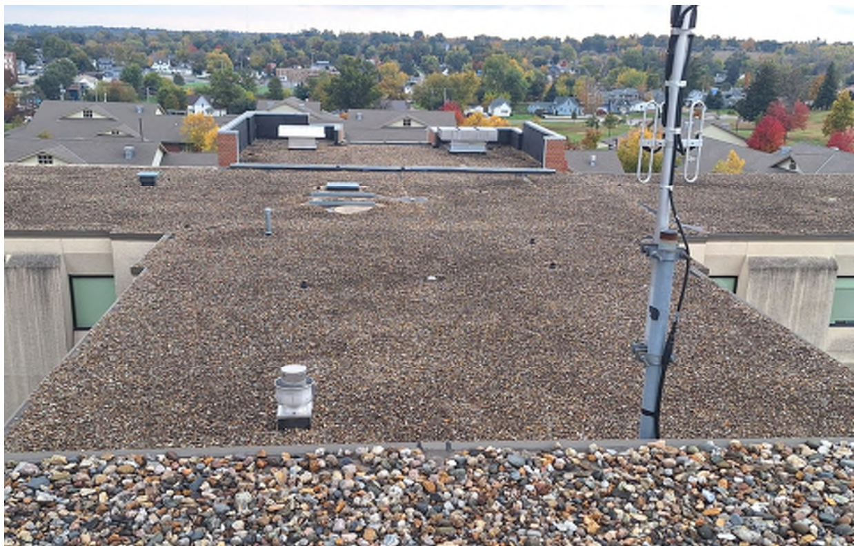
MALLOY ROOF - SOUTH ENTRANCE VIEWED FROM PENTHOUSE
