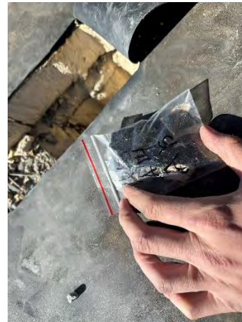
Photo #4 Sample A-14 Black Tar Roof Buildup around Perimeter, Malloy Building ( 30% Chrysotile )
