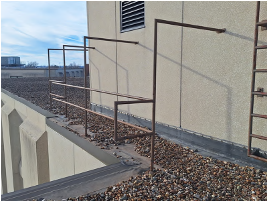
DACK ROOF - SOUTH GUARDRAIL
