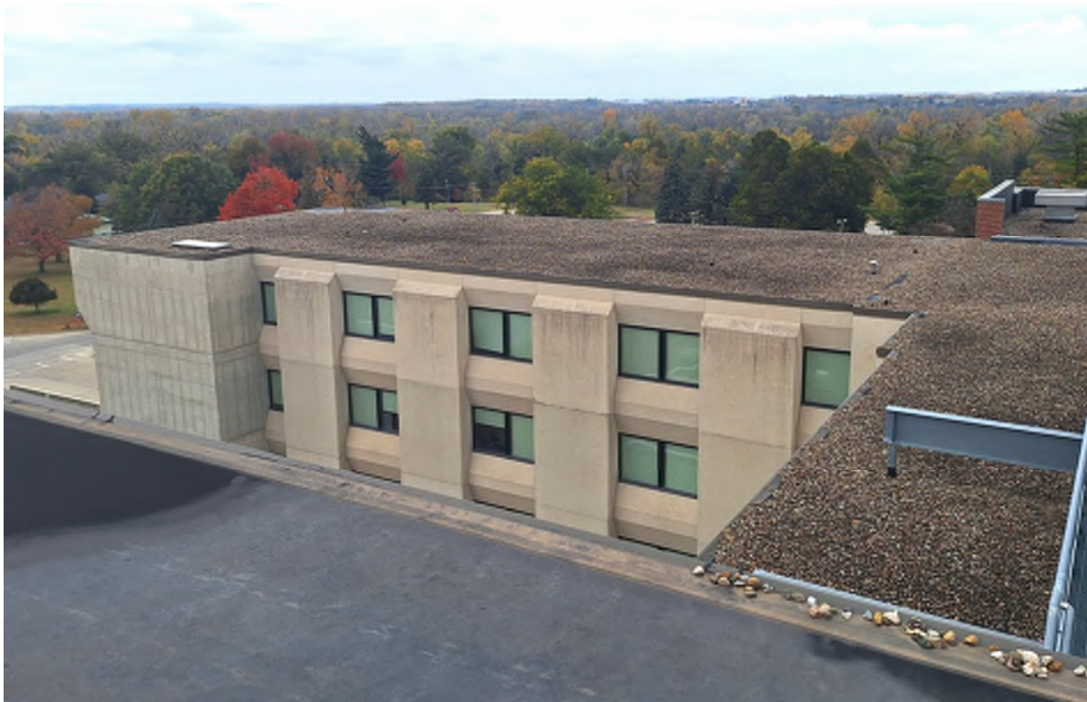
MALLOY ROOF - NORTHWEST WING
