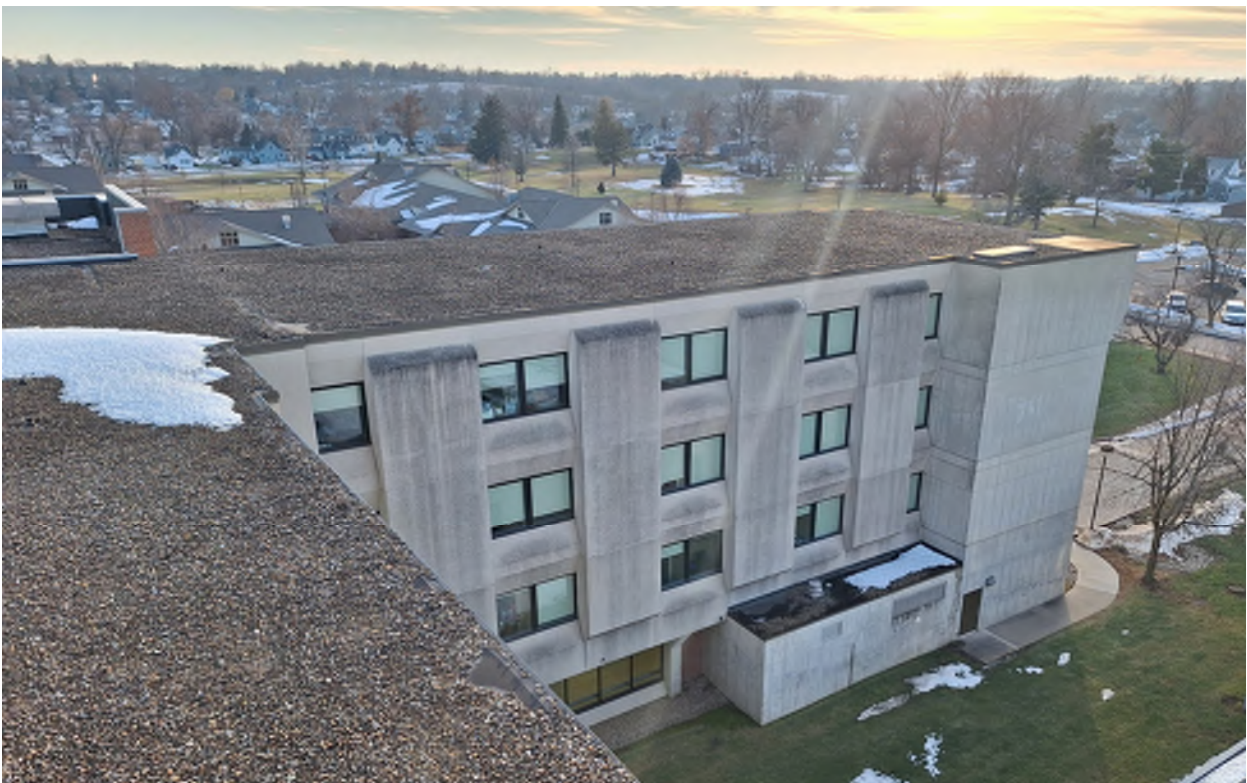
MALLOY ROOF - SOUTHWEST WING & LOWER ROOF
