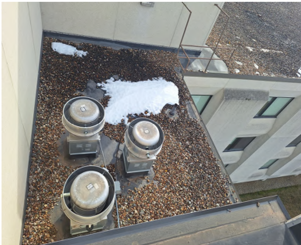
DACK ROOF - EXHAUST VENTS AT NORTH CORNER
