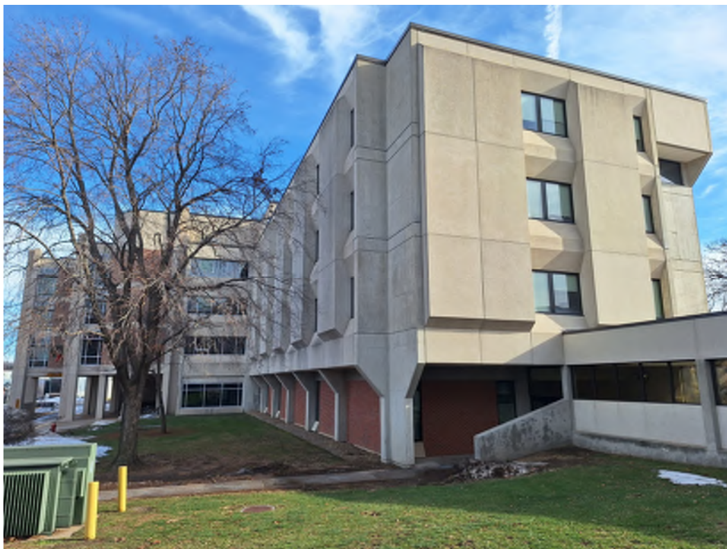
DACK BUILDING EXTERIOR - WEST END AND CORRIDOR LINK
