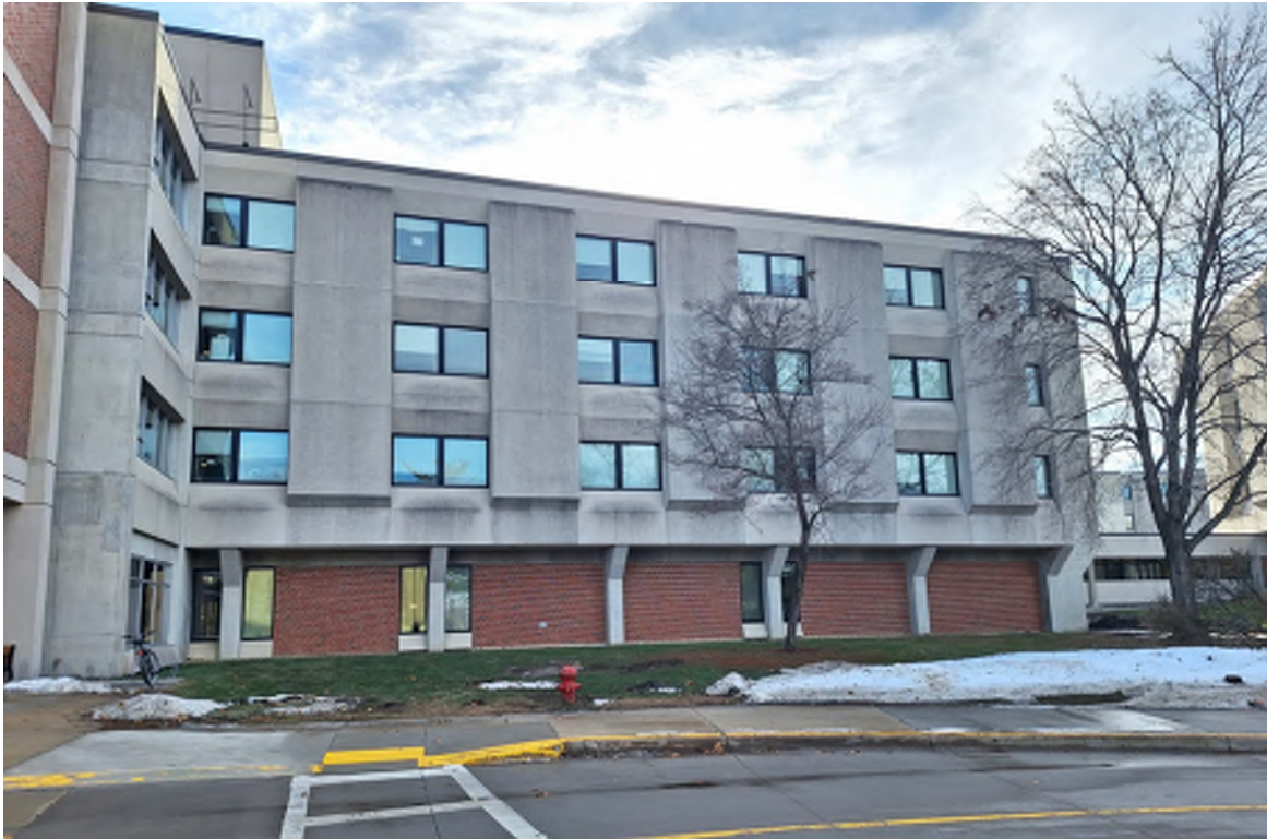
DACK BUILDING EXTERIOR - NORTHWEST ROOF ACCESS AREA
