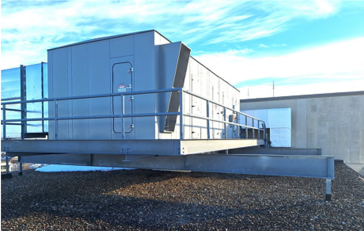
MALLOY ROOF - RTU SUPPORT BEAMS
