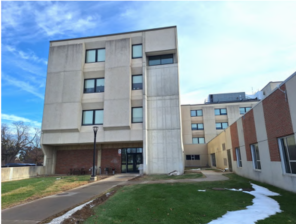
MALLOY BUILDING EXTERIOR - NORTHWEST ROOF ACCESS AREA
