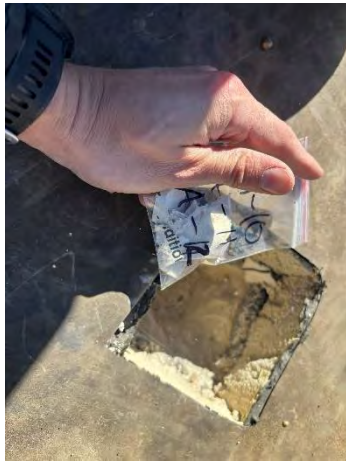
Photo #3 Sample A-12, 18, 27, 34 Black Roof Tar, Malloy Building Northwest Central ( 5-20% Chrysotile )
