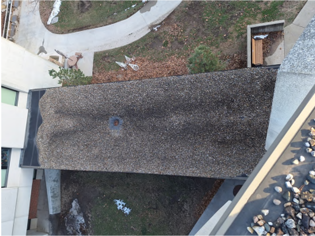
DACK-MALLOY CONNECTING COORIDOR ROOF
