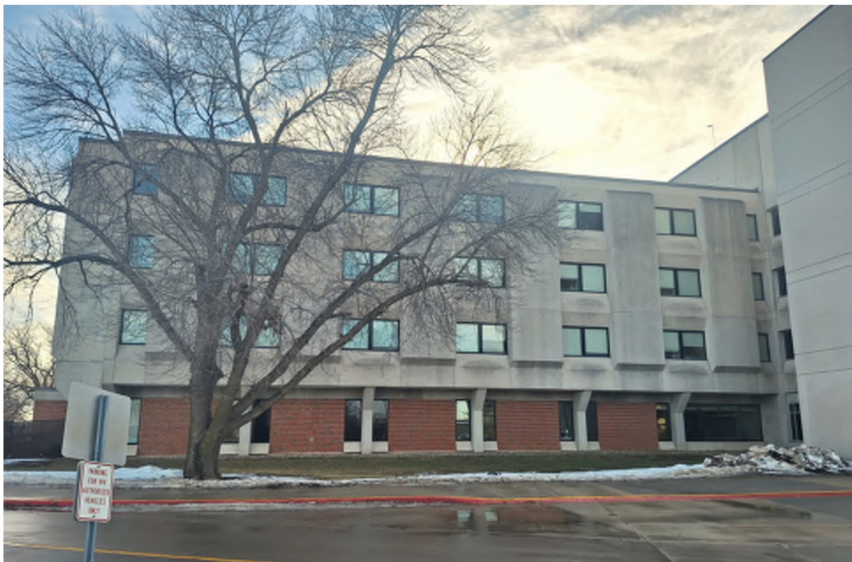
DACK BUILDING EXTERIOR - NORTHEAST ROOF ACCESS AREA
