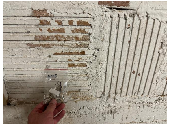
Photo #4 Lead-based paint on brick wall in basement (Sample DPPB-4).
