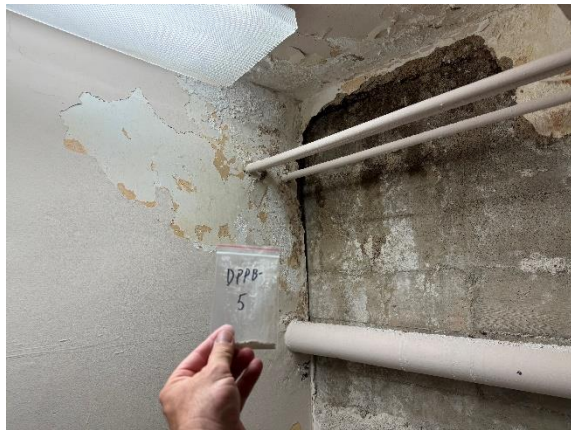
Photo #3 Lead-based paint on concrete wall in basement (Sample DPPB-5).
