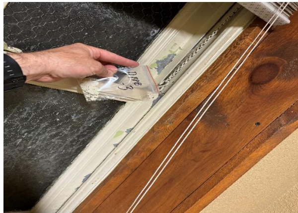
Photo #5 Lead-based paint on window in restroom (Sample DPPB-3).
