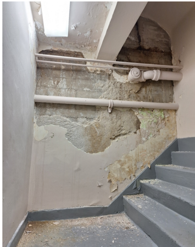
BASEMENT PLASTER REPAIRS
