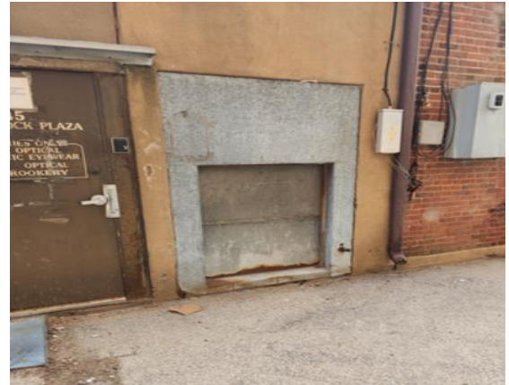
Photo #6 Asbestos black caulking around chute door (Sample DPPB-18).
