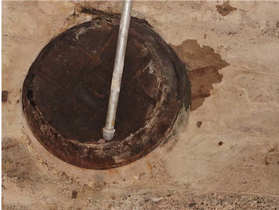
MANHOLE FOR INFILL IN CONCRETE LID
