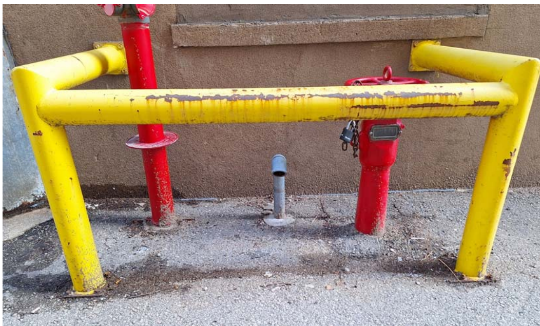
SPRINKLER PIPES & BOLLARD STANCHION
