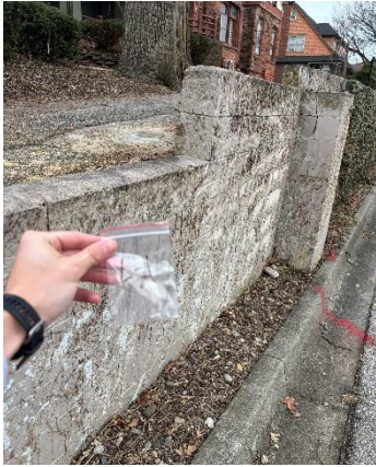
Photo #1 Sample L-1 SE Retaining Wall Brown paint on Brick (no lead-based paint).
