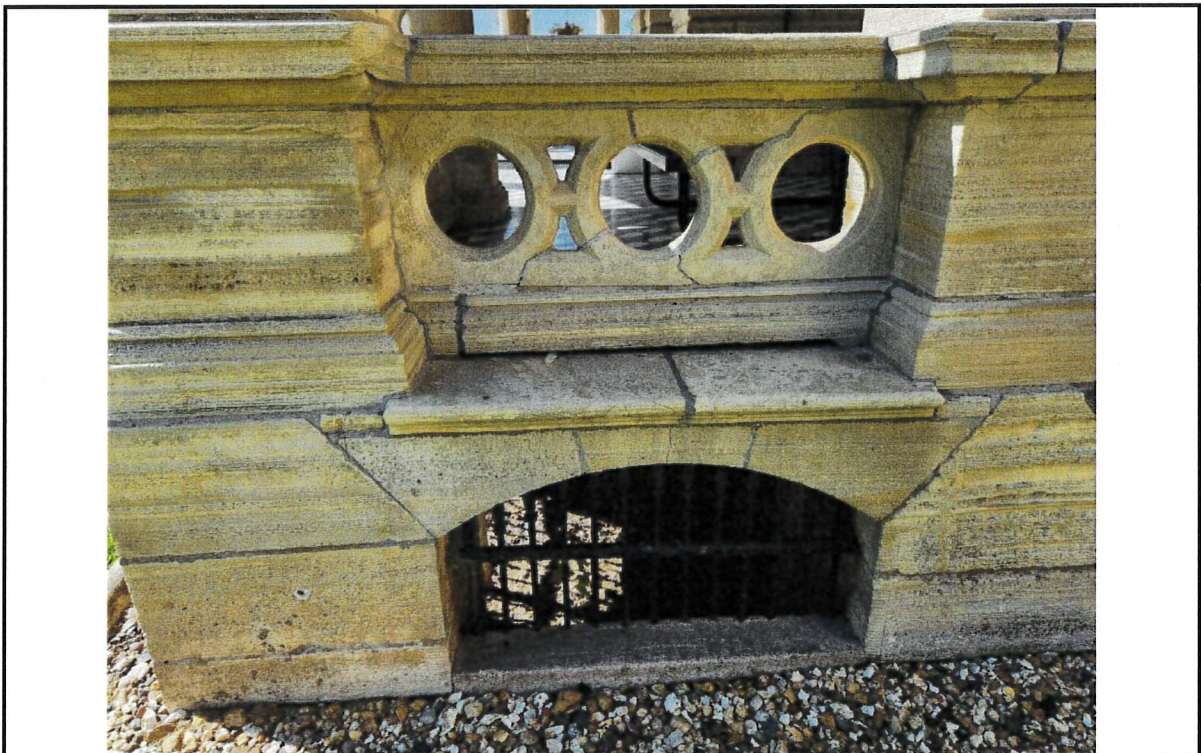
Photo 4: View of southeast portion of front of porch.
