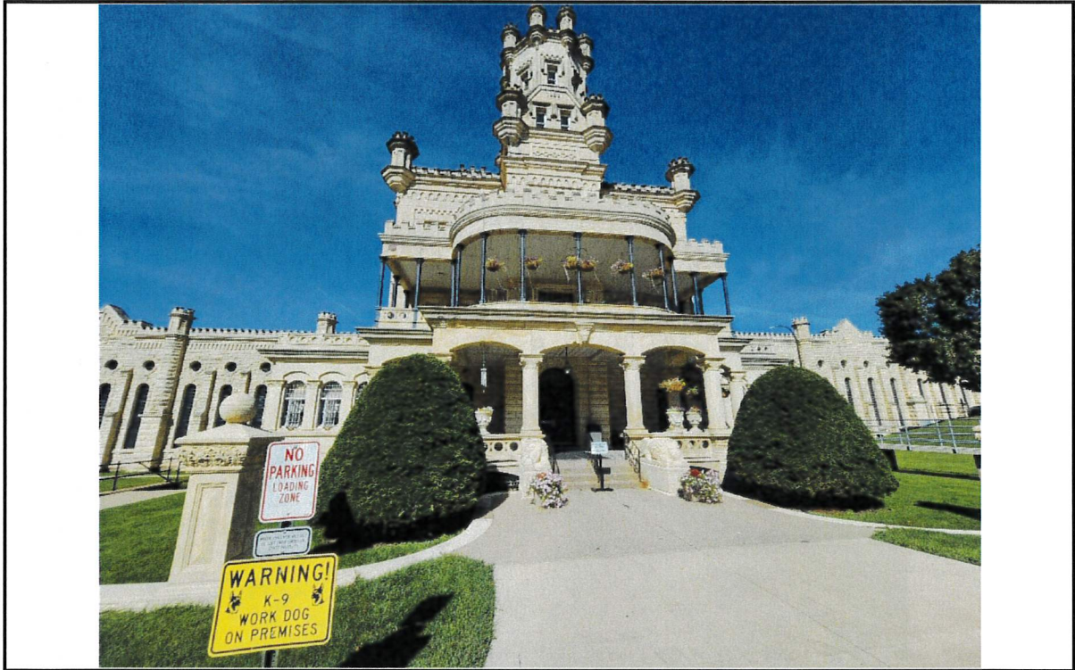
Photo 1: View of front of building and front porch
