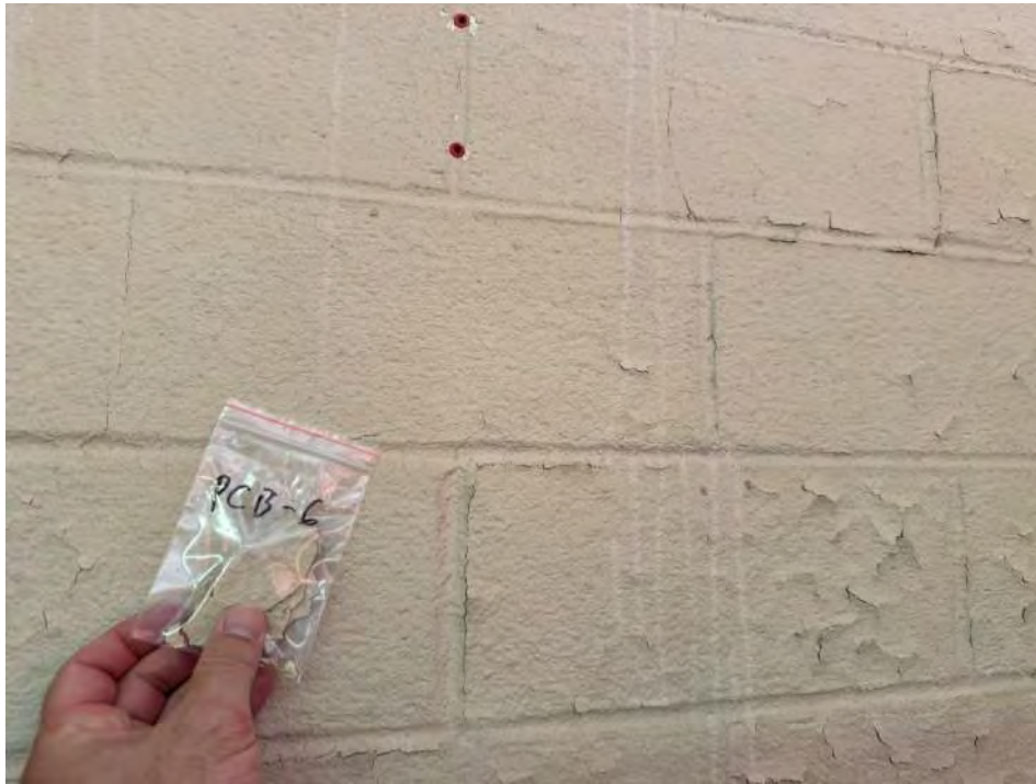
View of the Cream/Tan Lead Containing Paint. (PCB-6, 0.013% Pb)
