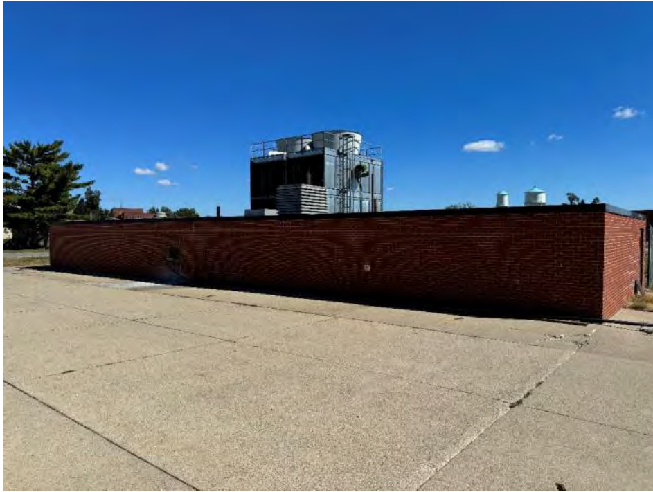
View of the Chiller Building.
