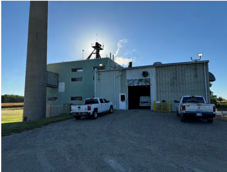
View of the Powerhouse.
