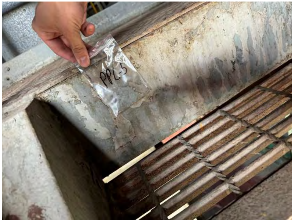
View of the Gray Lead Containing Paint. (PC-5, 0.034% Pb)
