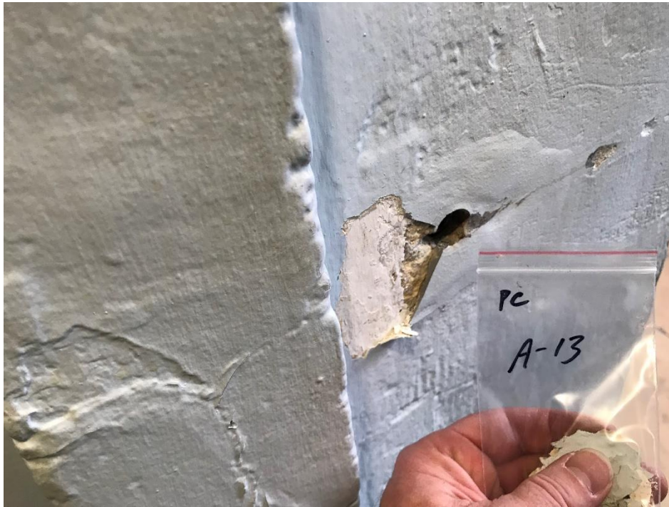
View of the light Blue Lead Containing Paint on Door Frame (PC A-13, 0.14% Pb).
