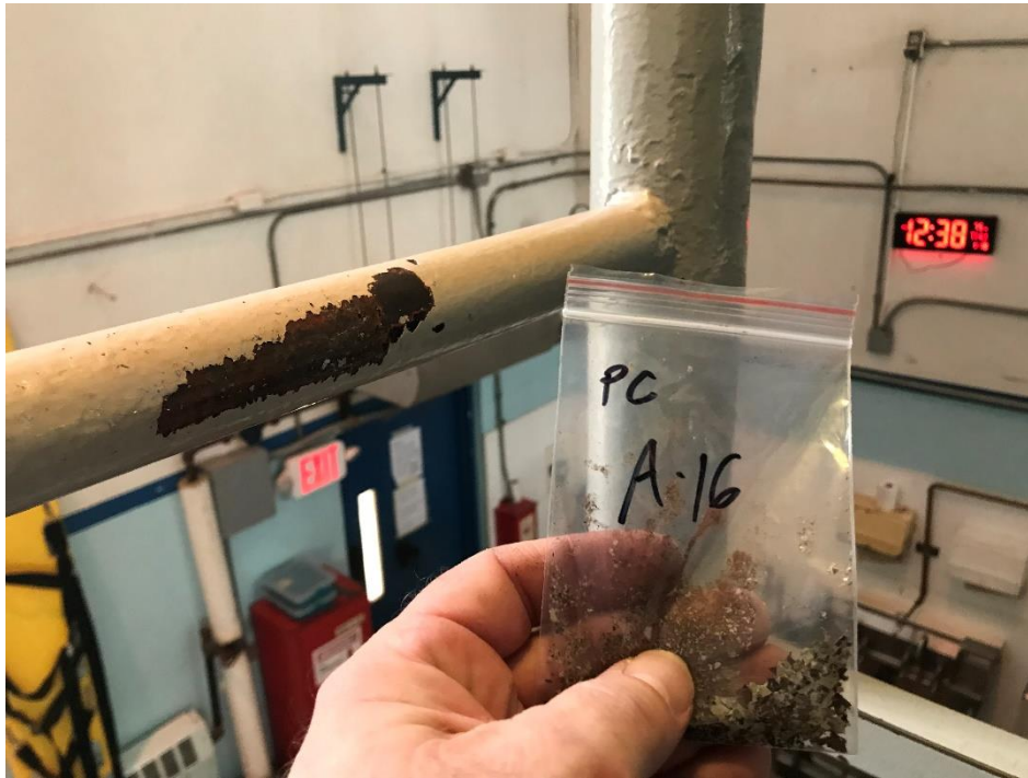
View of the Beige/Gray Lead Containing Paint on Handrails (PC A-16, 0.008% Pb).
