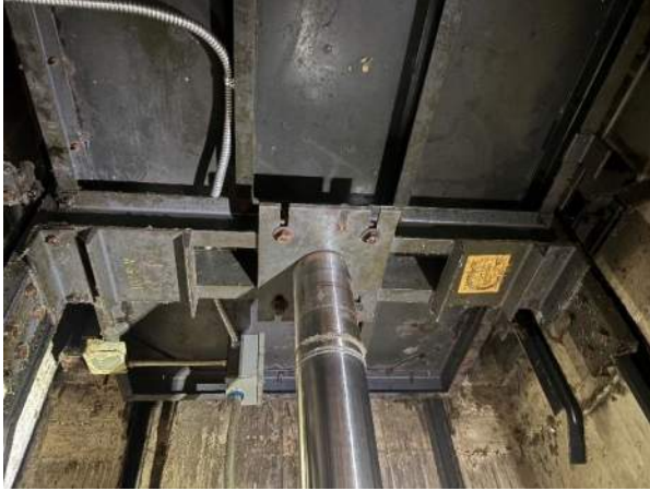
Photo #1 Bottom of Food Service Elevator
