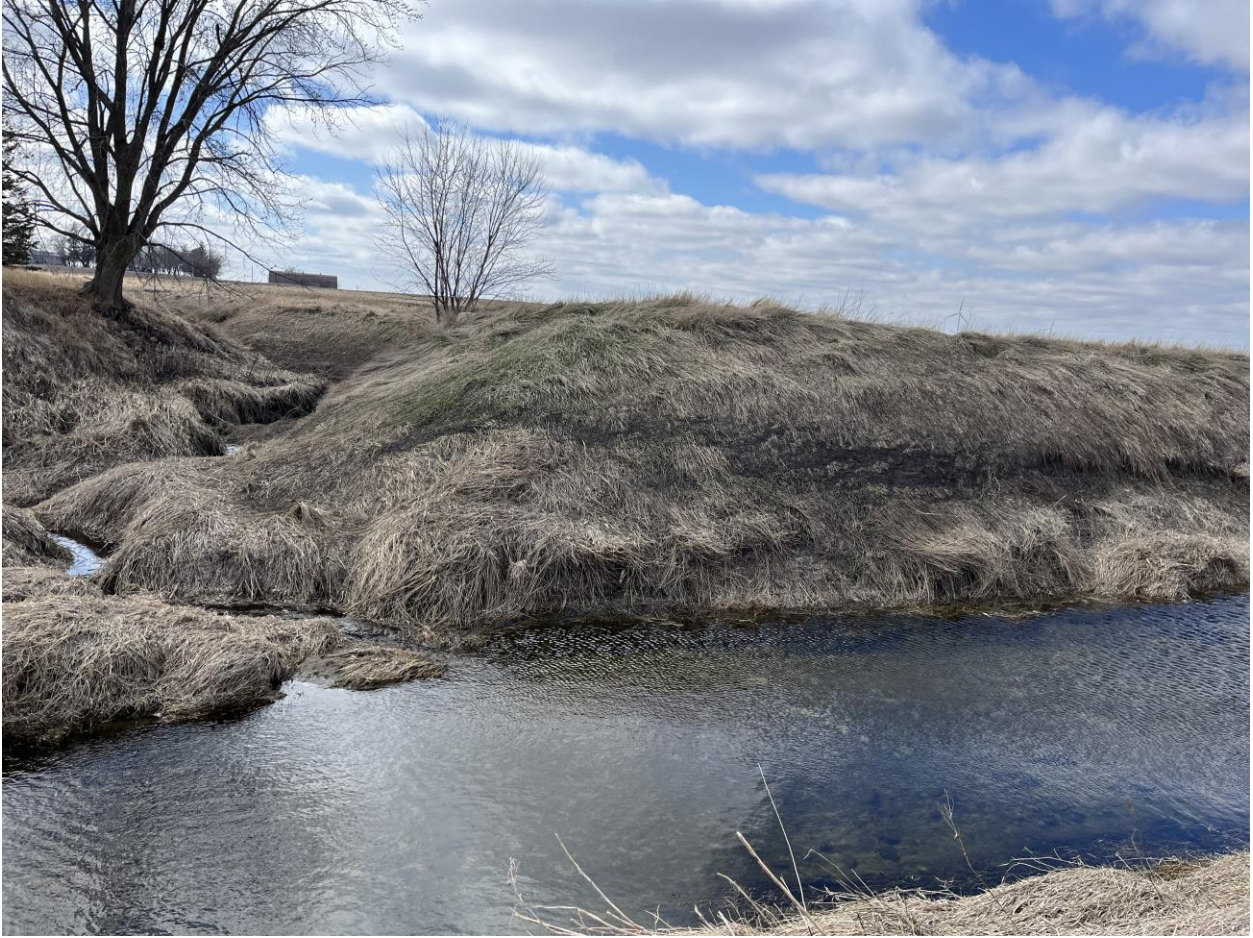
Channel outlet area into Lizard Creek (looking west)
