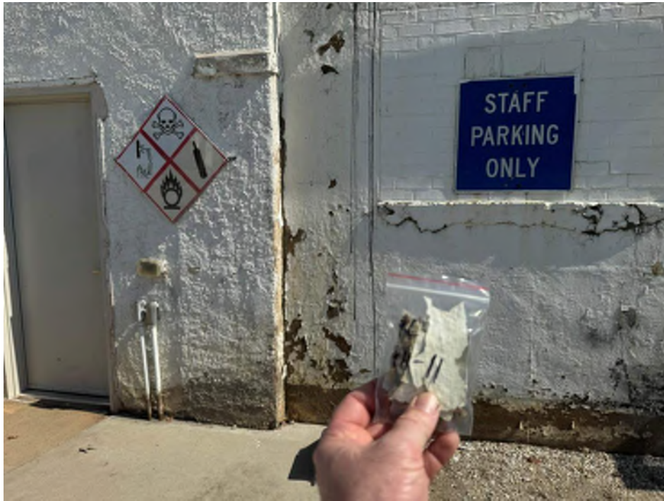
View of the Lead Containing White Paint. (Powerhouse Sample: PC PH-11, 1.4% Pb)
