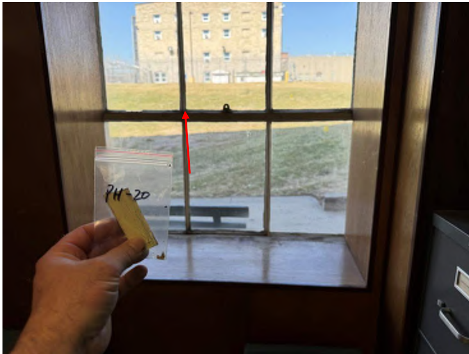
View of the Powerhouse Window Glazing. (Sample PH-20, 3% Chrysotile)
