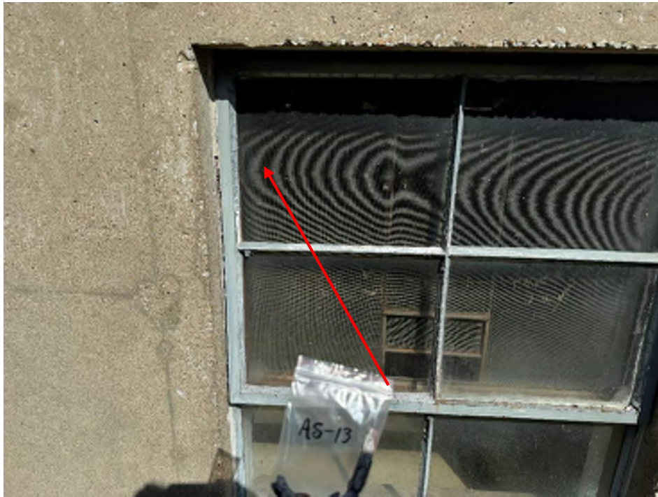
View of the Appliance Shop Gray Caulk. (Sample AS-13, 4% Chrysotile)
