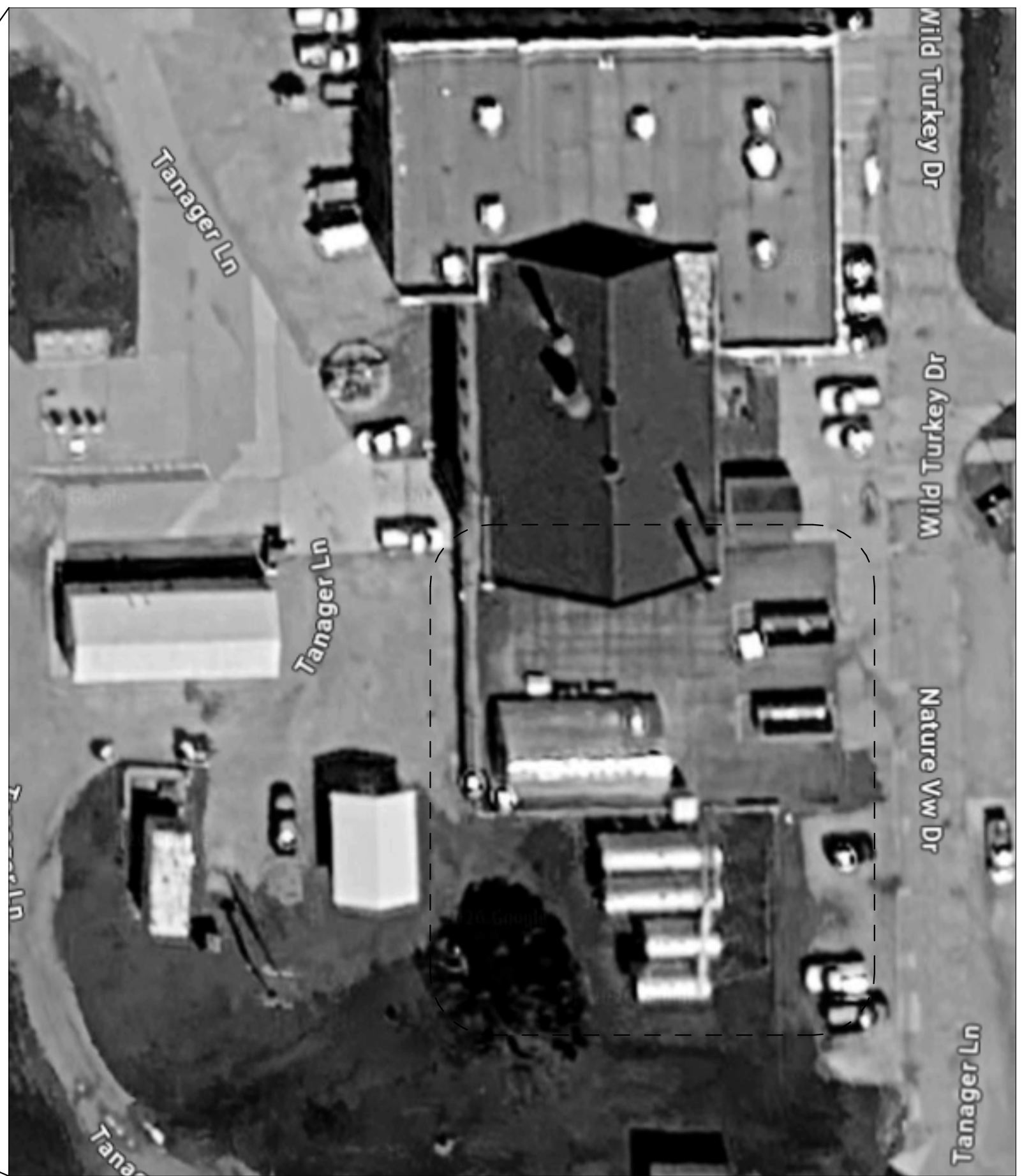
PLANT BASEMENT ROOF AND DIESEL TANKS
