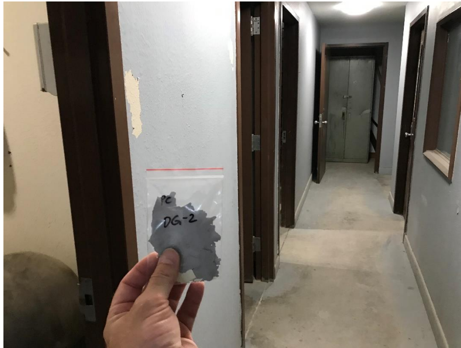
Paint chip sample #2 from the wall in the office hallway.
