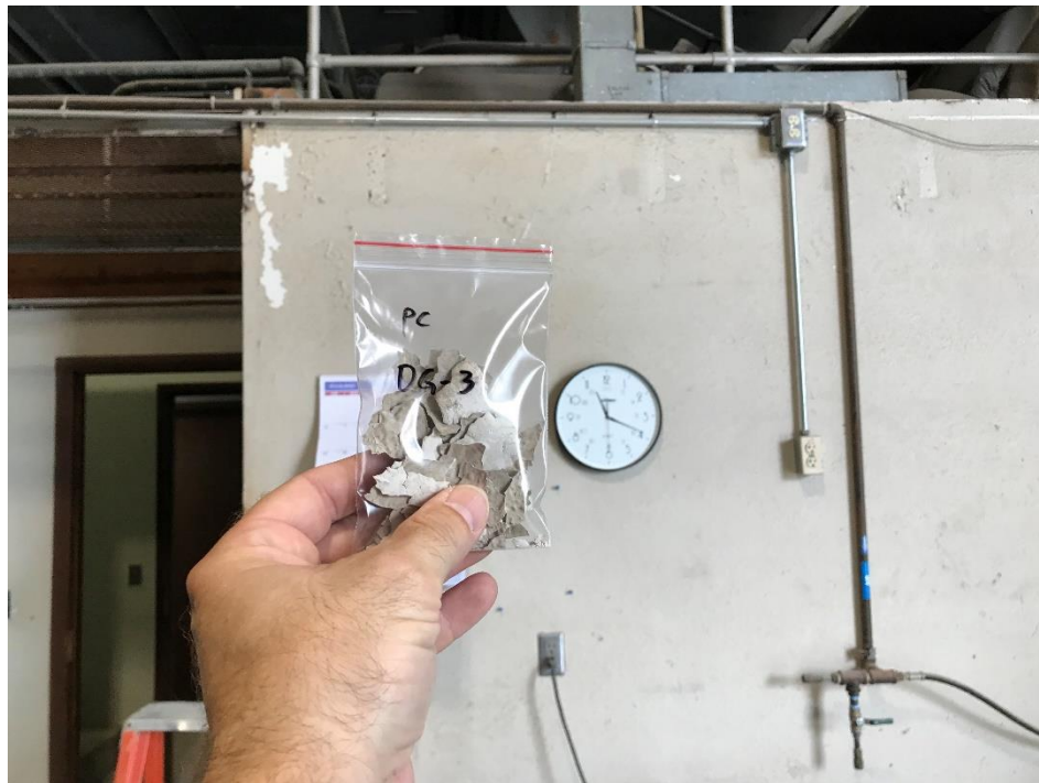
Paint chip sample #3 from wall in the garage.
