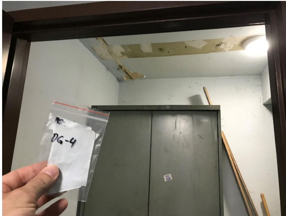
Paint chip sample #4 from office closet ceiling.
