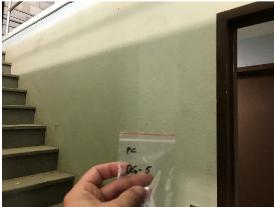
Paint chip sample #5 from wall in stairway.
