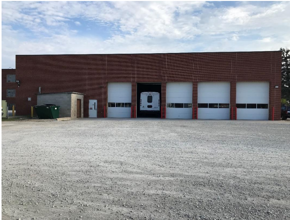
Looking North at Dispatch Garage.
