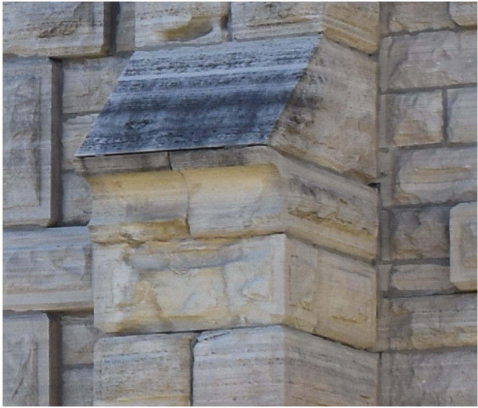
TYPICAL CONDITION REQUIRING CONSOLIDATION PER KEYNOTE 6
