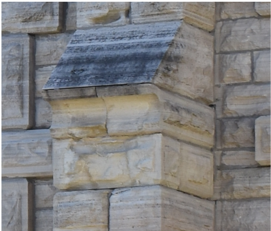
TYPICAL CONDITION REQUIRING CONSOLIDATION PER KEYNOTE 6
