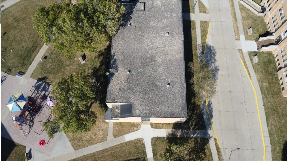
DOE ISD Elementary School Roof Replacement Design RFP945600-01
