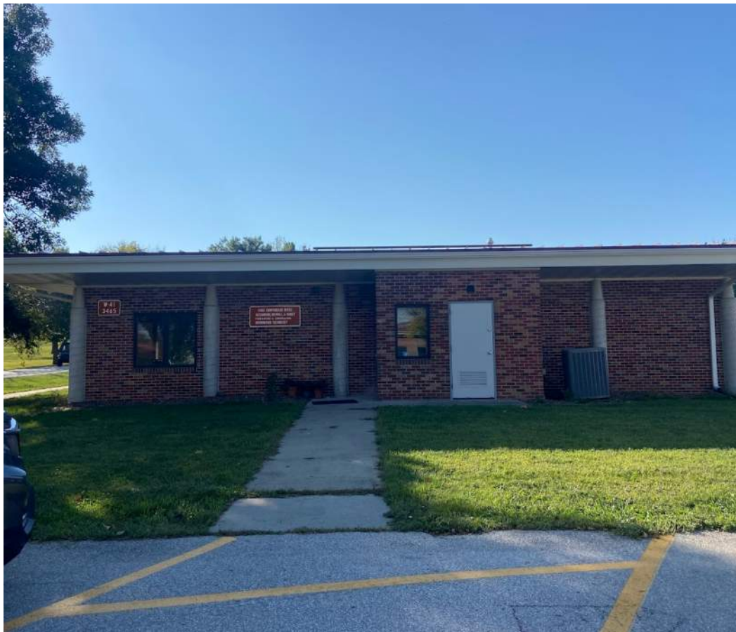
Photo 2: North elevation of the building looking south
