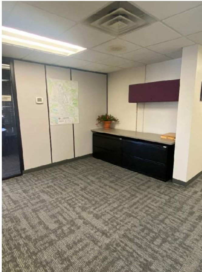
Photo 14: Sloped slab north of room 117
