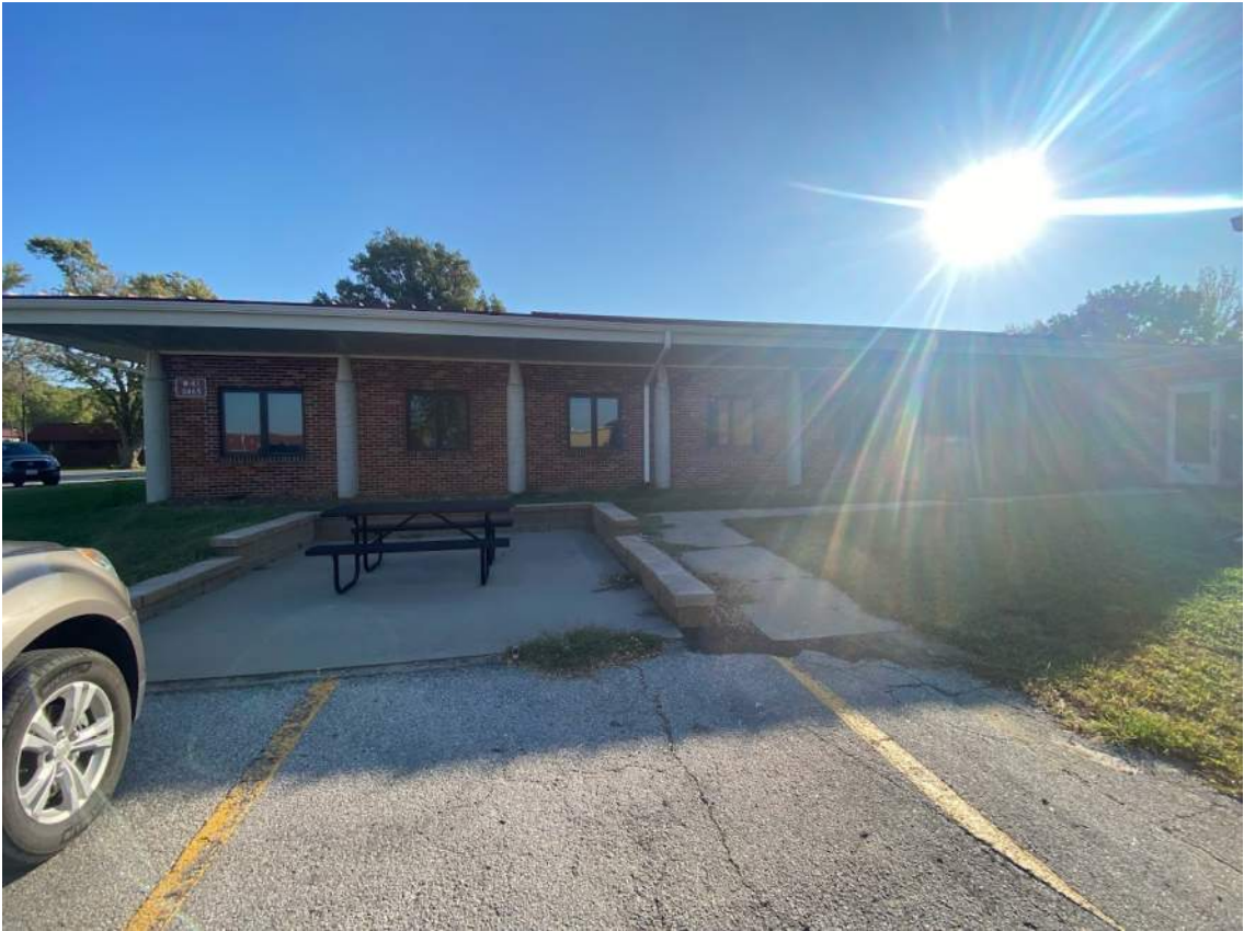
Photo 5: North-west elevation of the building looking east
