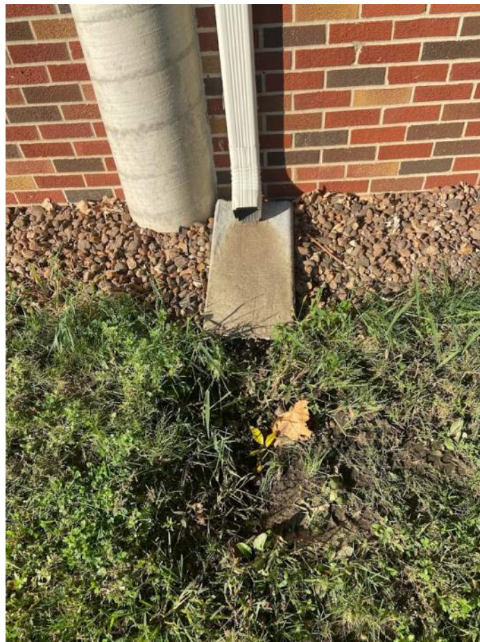
Photo 6: Typical downspout with splash block
