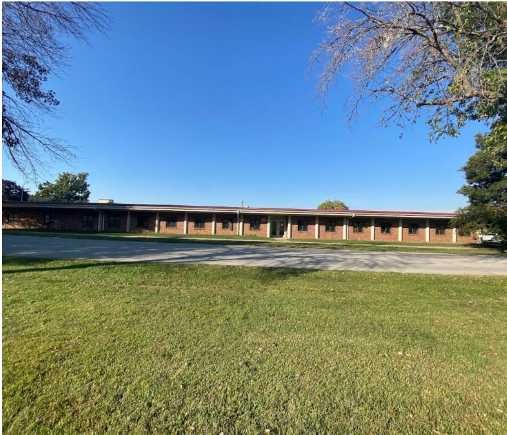
Photo 1: East elevation of the building looking west
