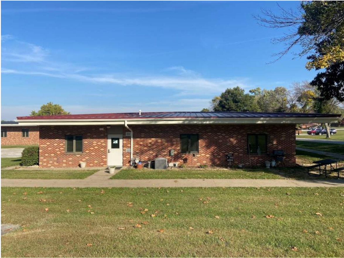
Photo 3: South elevation of the building looking north
