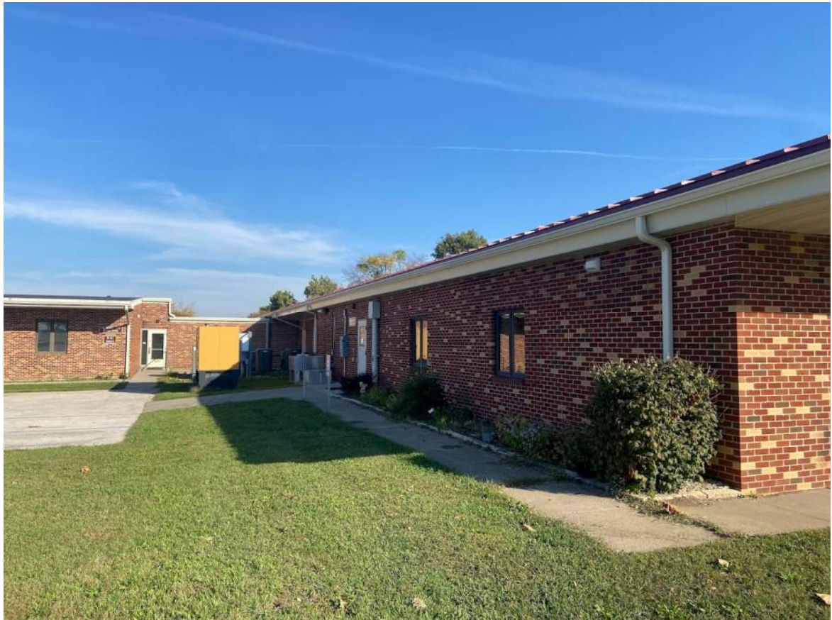
Photo 4: South-west elevation of the building looking north
