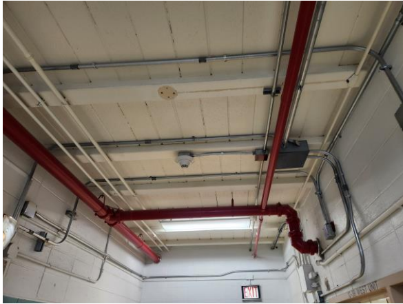
Photo #7 Corridor between SNU and Main East and West.
