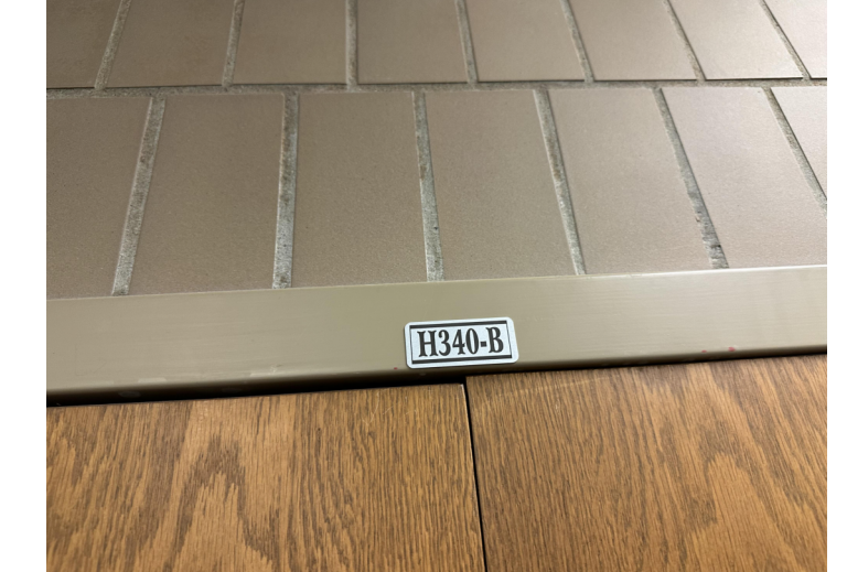
* NEW SIGNAGE TO MATCH EXISTING (MATERIAL, SIZE, FONT, ETC). SEE PHOTO ABOVE FOR REFERENCE.
